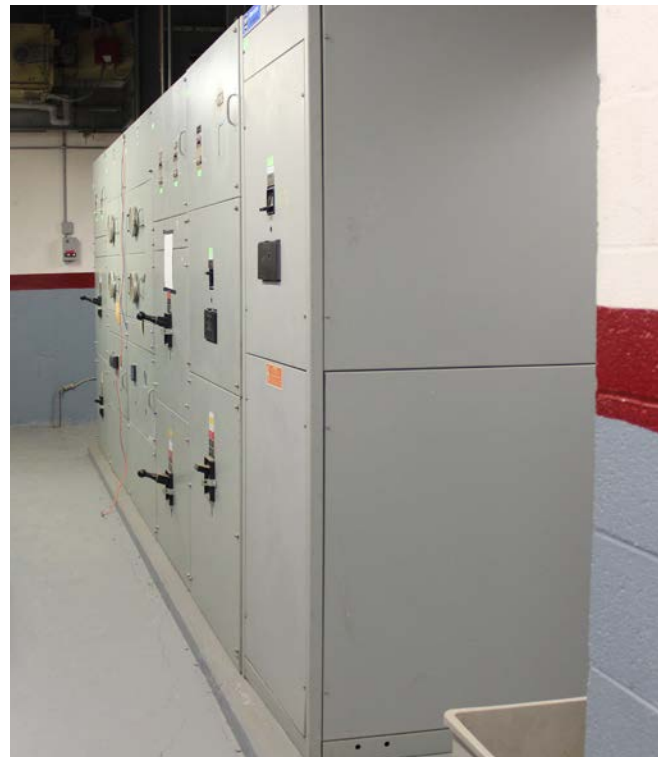
Selection of existing MEP Infrastructure
