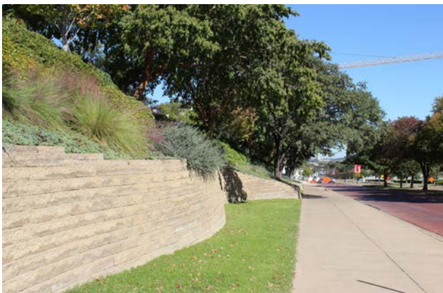
Retaining Walls Exist at Multiple Places on Campus to Hold Back Earth Elements
