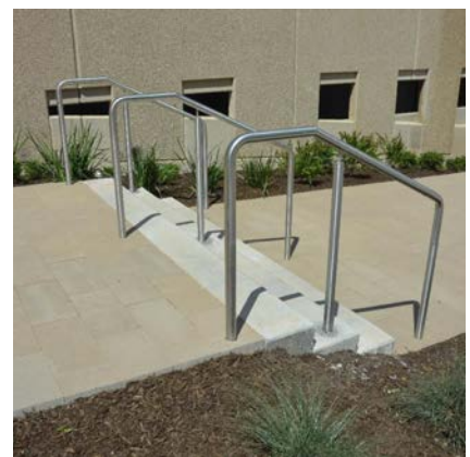
Stair Railings Existing on campus
