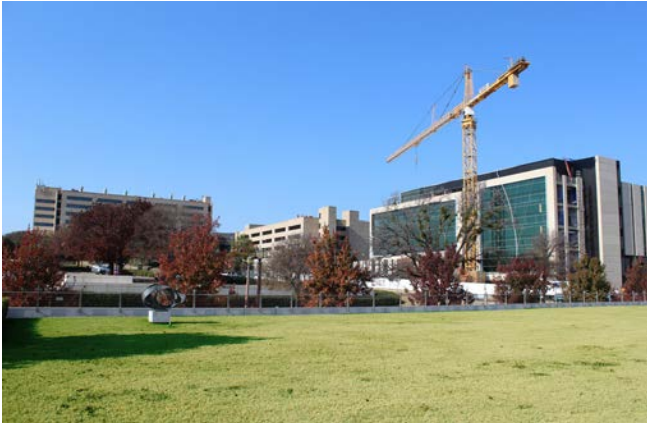
2. View to Campus from Kimbell Pavilion Roof
