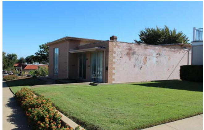
Facilities Support Annex, Constructed in 1965 Differing Exterior Character and Quality
