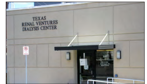
Building Identification - Building Facade
