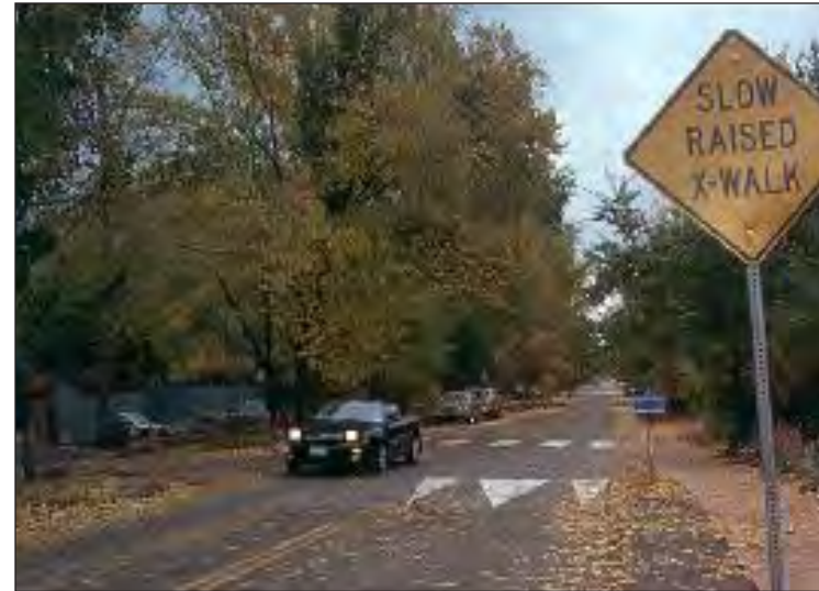
Speed tables or raised crosswalks reduce vehicular traffic, improve crosswalk visibility and enhance the environment for pedestrians
