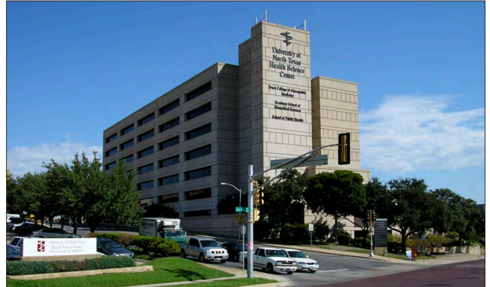
Existing front door at Montgomery Drive and Camp Bowie Boulevard
