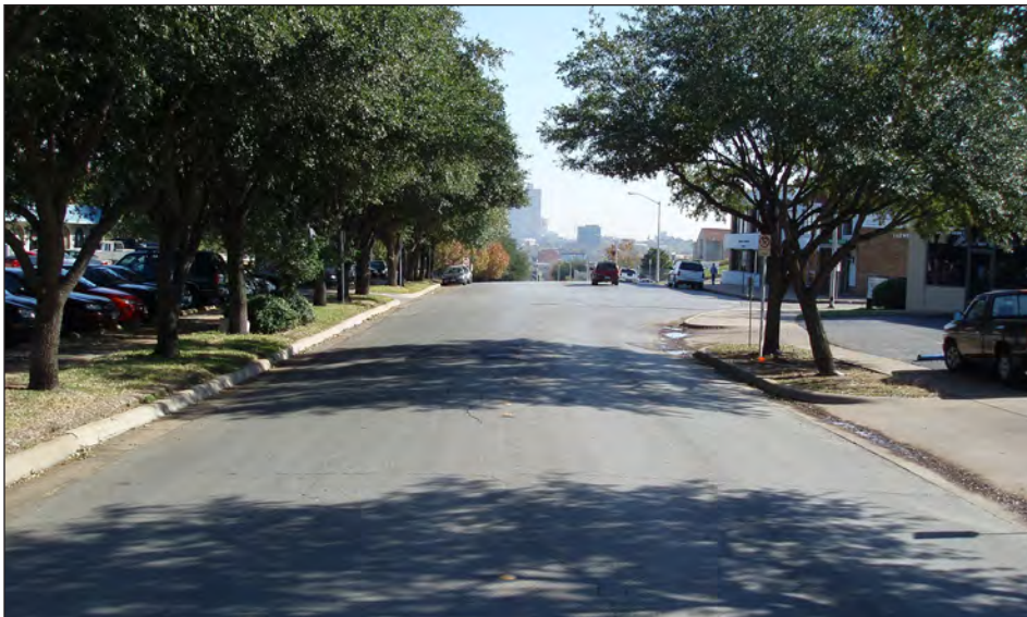
7 th and Montgomery - Looking East
