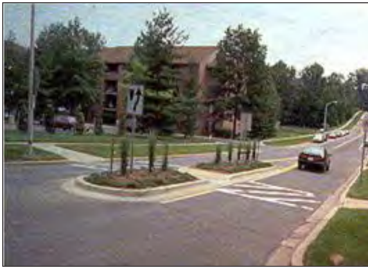
Additional example of roadway narrowing
