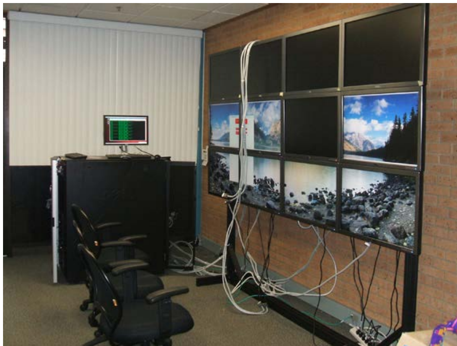
Popcorn anyone? Currently under construction, the RAVE video wall will allow researchers to view their data on a grand scale
