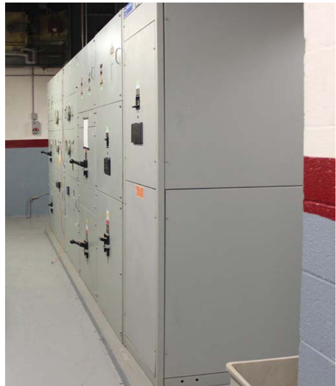
Selection of existing MEP Infrastructure
