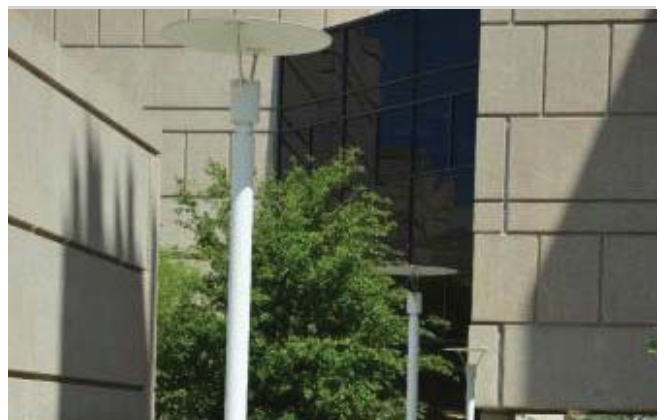
BEGA Pedestrian Lights Existing on campus
