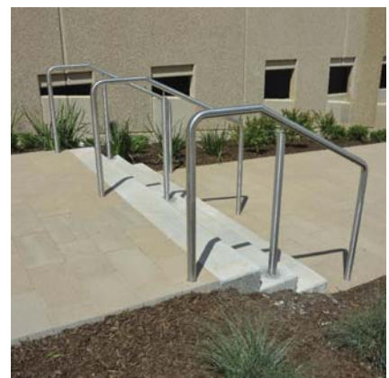
Stair Railings Existing on campus
