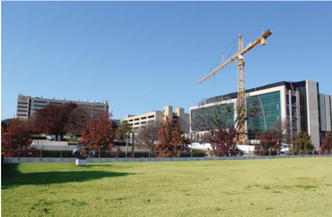
2. View to Campus from Kimbell Pavilion Roof
