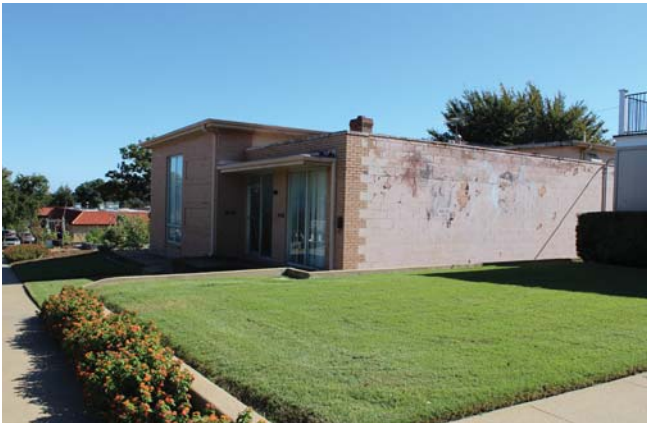
Facilities Support Annex, Constructed in 1965 Differing Exterior Character and Quality
