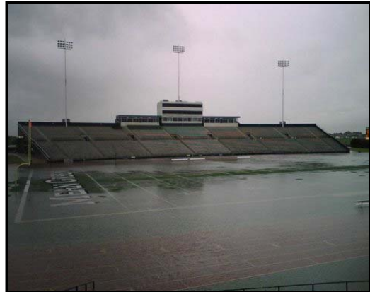
Figure 5: A spring storm caused flash flooding at Fouts Field in 2007
