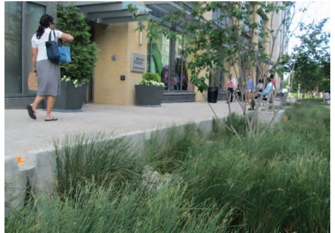
Low-Impact Development - Bioswale
