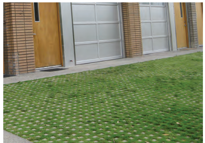
Low-Impact Development - Permeable Pavement
