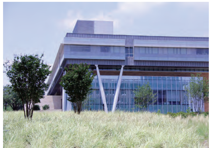
Sustainable Building Design- UNT
