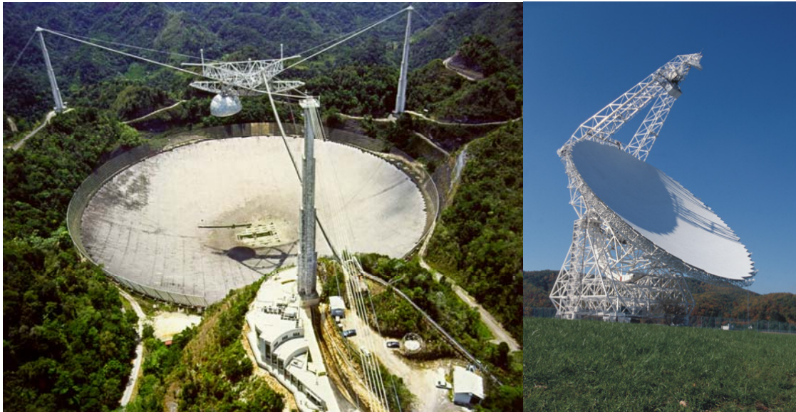
Figure 11. (a) On the left is the 300m diameter Arecibo telescope in Puerto Rico operated from 3 MHz to 10 GHz by NAIC. A powerful radar and laser facility is used to probe solar system objects and the Earth's atmosphere. On the foreground hill is the popular Angel Ramos Visitor and Educational Center. [Image credit: NAIC] (b) On the right is the Robert C. Byrd Green Bank Telescope at Green Bank, WV, the world's largest fully steerable, single-dish antenna. Current observations extend from 290 MHz to 52 GHz and will eventually extend into the 95-GHz atmospheric window. Green Bank is centered in the National Radio Quiet Zone that provides considerable protection from man-made interference. [Image credit: NRAO/AUI]
