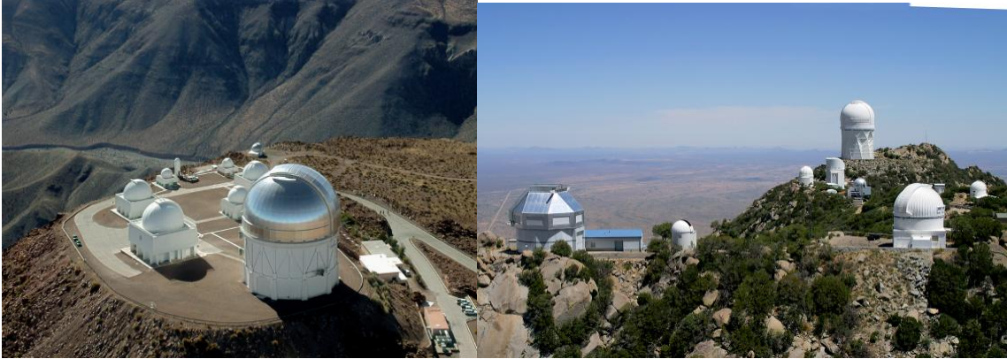
Figure 10. (a) On the left is the CTIO site that is managed by NOAO in Chile. The large dome in foreground holds the Blanco 4m optical telescope. Four smaller domes near the Blanco contain 1.5m, 1.3m, 1.0m and 0.9m optical telescopes operated as the Small and Moderate Aperture Research Telescope System (SMARTS) led by Yale University in cooperation with NOAO. (b) The large dome on the right contains the Mayall 4m optical telescope operated by NOAO at the KPNO site outside Tucson, Arizona. The nearer dome on right is the KPNO 2.1m telescope. The intervening domes hold University of Arizona Steward Observatory telescopes. The multi-faceted dome on the left holds the 4m Wisconsin-Indiana-Yale-NOAO (WIYN) 4m optical telescope. Adjacent to WIYN's lab building is their 0.9m telescope. [Image credit: NOAO/AURA/NSF]
