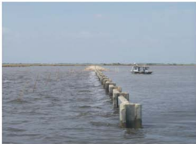
Concrete "H" pile/panel structures, similar to this one, will be installed at locations within the project area where shoreline erosion is critical. Soils with high amounts of organic material, which have poor strength, necessitated the use of a structure such as this.
