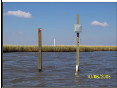
Figure 4: CRMS0375 continuous recorder and staff gauge post. Notice vegetation around the electrical box.
