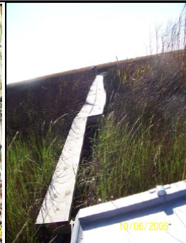
Figure 2: CRMS0434 boardwalk with missing board and warning sign post.
