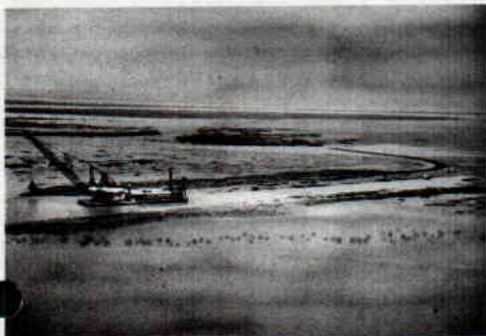
This restoration technique is an example of what is proposed in the Castille Pass.
