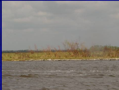
No shoreline erosion due to Hurricanes Katrina and Rita – protection feature part of Jonathan Davis Wetland Project (BA-20).
