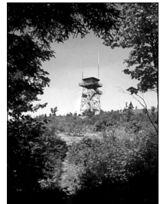
Ojibway Tower has housed air monitoring instrumentation since 1987.
