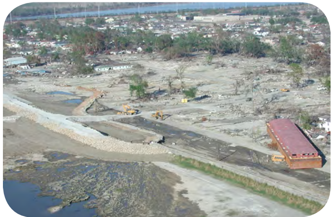
Figure 10. Panoramic view from the lift bridge seen in background in figure 9A. Note the barge on the right and the temporary levee repair by the U.S. Army Corps of Engineers.
