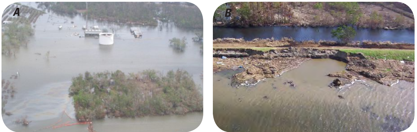
Figure 2. Complete levee failure at Nairn, La. (A), and partial failure with severe loss of cross section (B) as a result of Hurricane Katrina in 2005. Photographs are from Plaquemines Parish government and used with permission.
