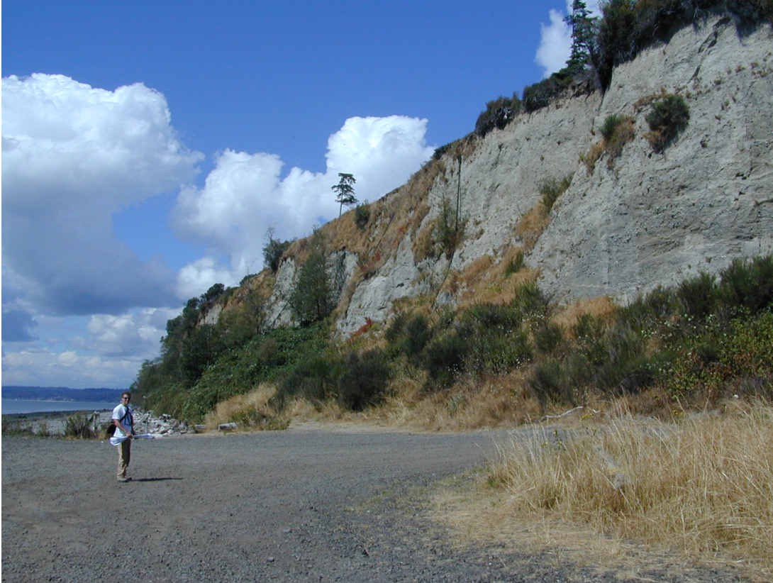
Figure 7. Typical nearly vertical coastal bluff with deposits of apparent falls and topples along bluff toe. The vegetated area at the base of the slopes roughly outlines the deposits of these failures. This picture was taken SW of Point Jefferson (landslide 24, see map) (photograph: Jeffrey A. Coe, 2003).
