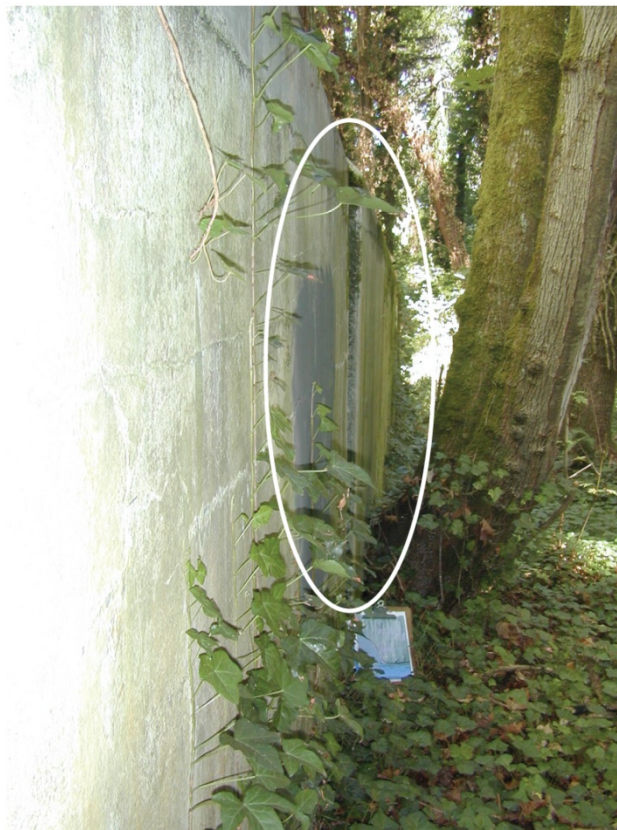
Figure 10A and 10B. Foundation of a gun battery located in a landslide scar (landslide 147, see map) at Fort Ward State Park on the south side of the Rich Passage. A ) Upper surface of the foundation. B ) Side view showing minor deformation, probably from settling of the foundation (photograph: Jeffrey A. Coe, 2003).
