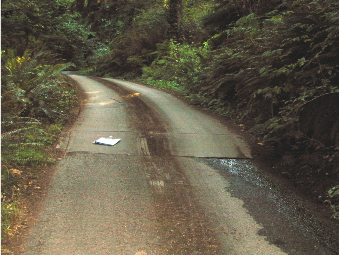
Figure 8. Asphalt-surfaced road offset along the headscarp of landslide 150 (see map) northeast of Bremerton. See clipboard for scale (photograph: Jeffrey A. Coe, 2003).
