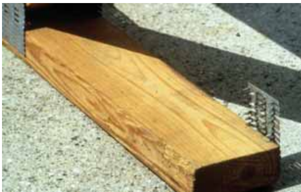
Figure C-2. Gusset plates. Note length of teeth/ penetration depth. (Photo courtesy of Vincent Dunn.)
