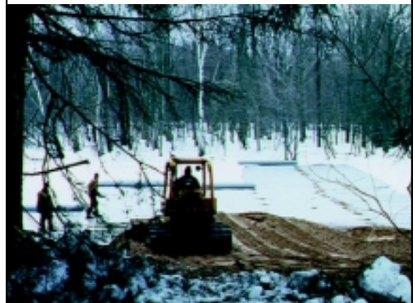
Figure 1. Spreading Geotextile over Frozen Lake
