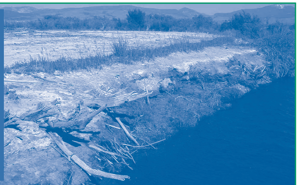
Figure 3. Remediation activities along the Clark Fork River will reflect RipES results with emphasis on those areas most in jeopardy of erosion into the river channel, such as this stream bank with active erosion.
