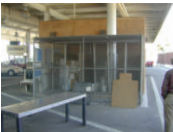
Kennel converted for outside storage
