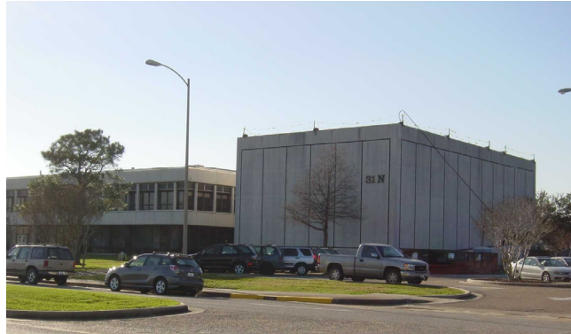
JSC Curation Building
