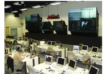
Range Control Center
