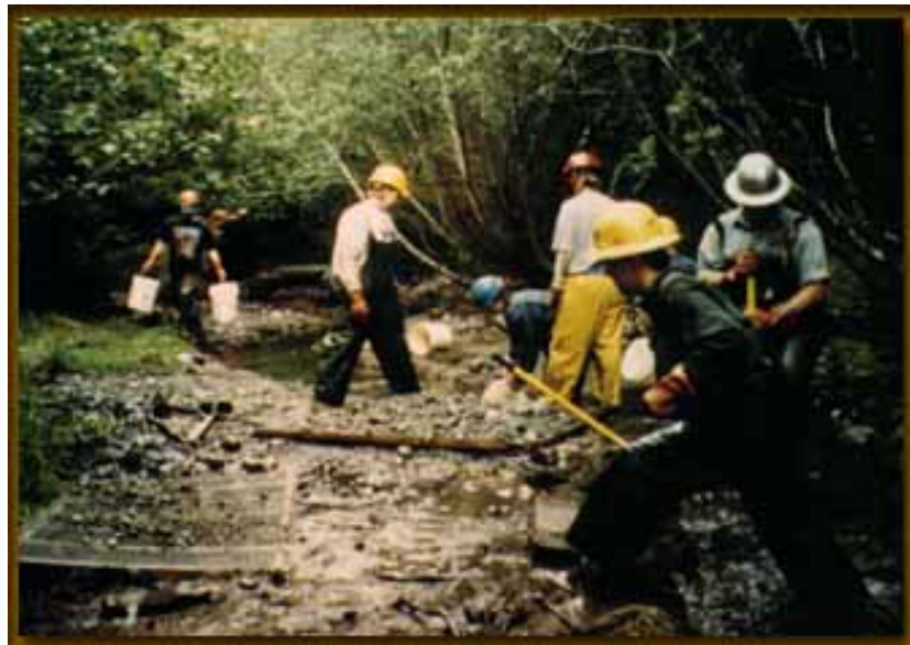
Americorps volunteers also used shovels and grates to manually remove fine sediment from degraded stream bed in order to improve spawning habitat.
