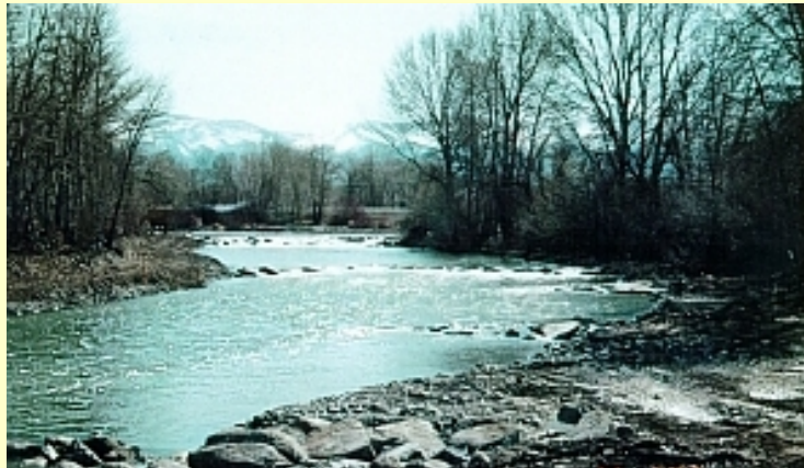
Vortex rock weirs, completed installation, Carson River, 1999
