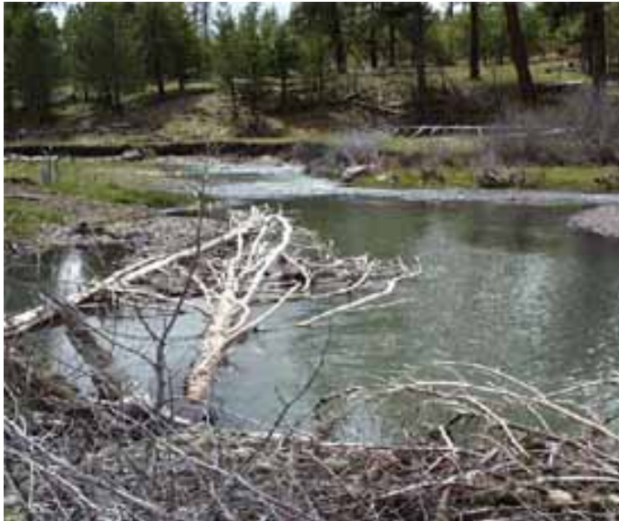
Figure 3: Woody debris was built into the design for McCoy Creek restoration to improve Salmon habitat.
