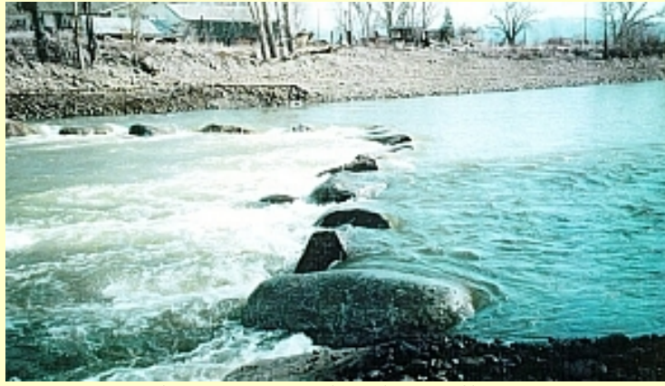
Vortex rock weirs, completed installation, Carson River, 1999
