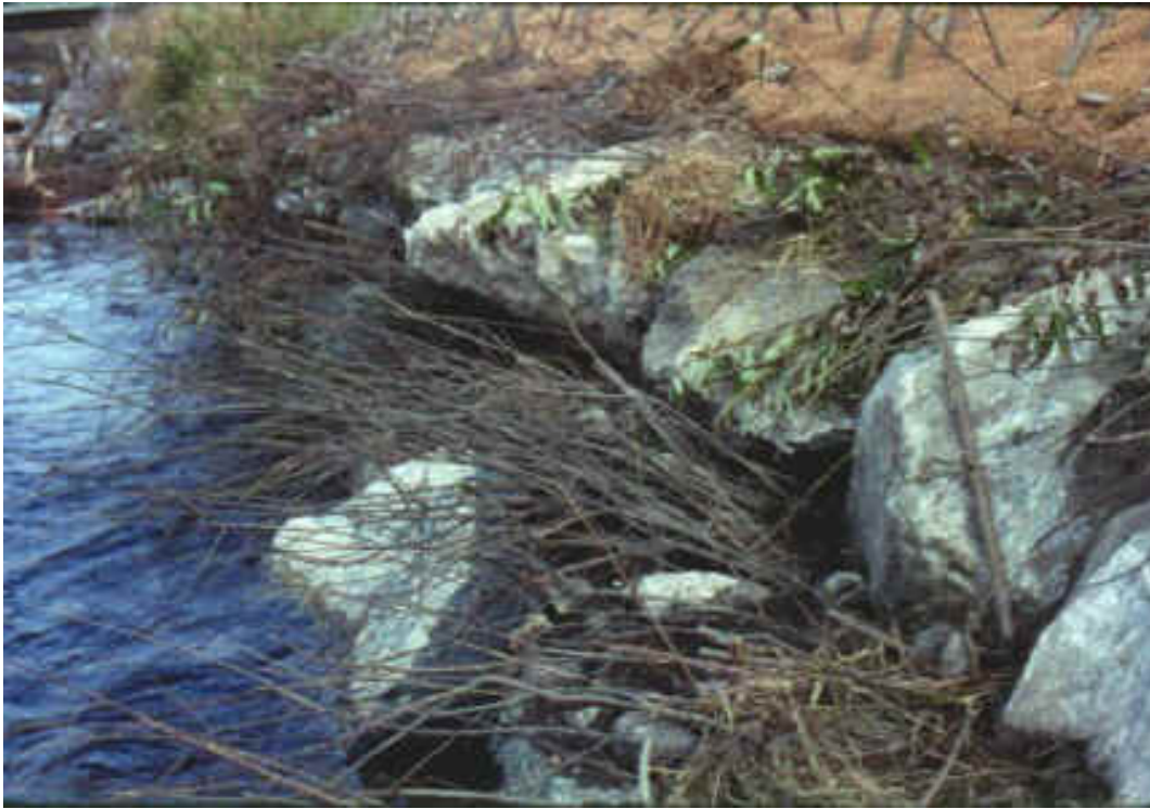
Close-up of rock revetment with brush layers
