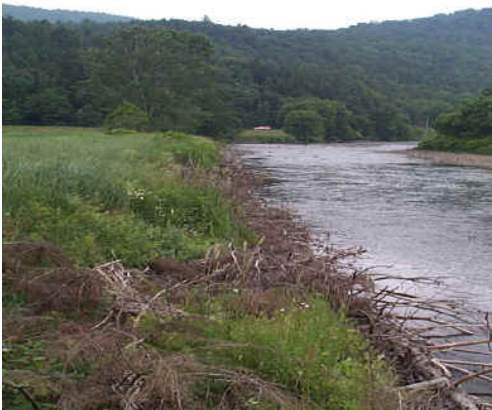
Tree revetments stabilizing toe of bank after 1 year
