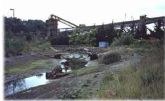
Lower Basin tidal marsh rehabilitation project.
