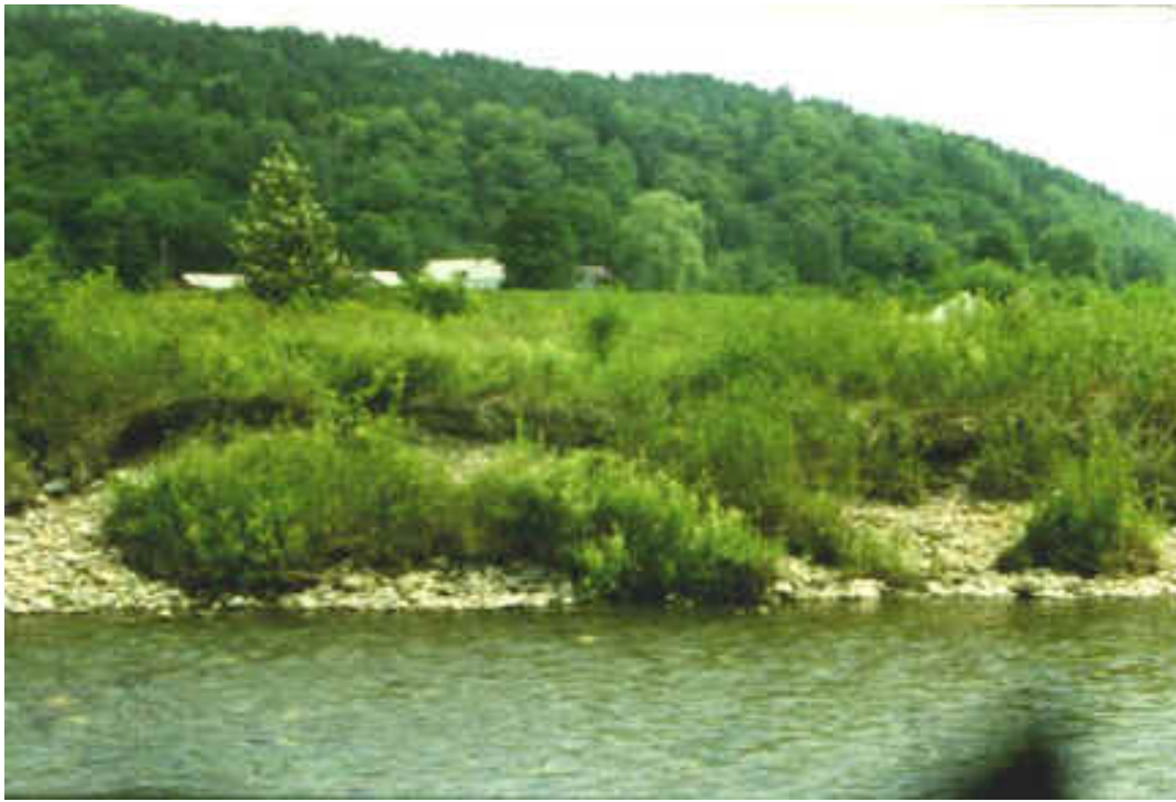
Slumping bank before treatment
