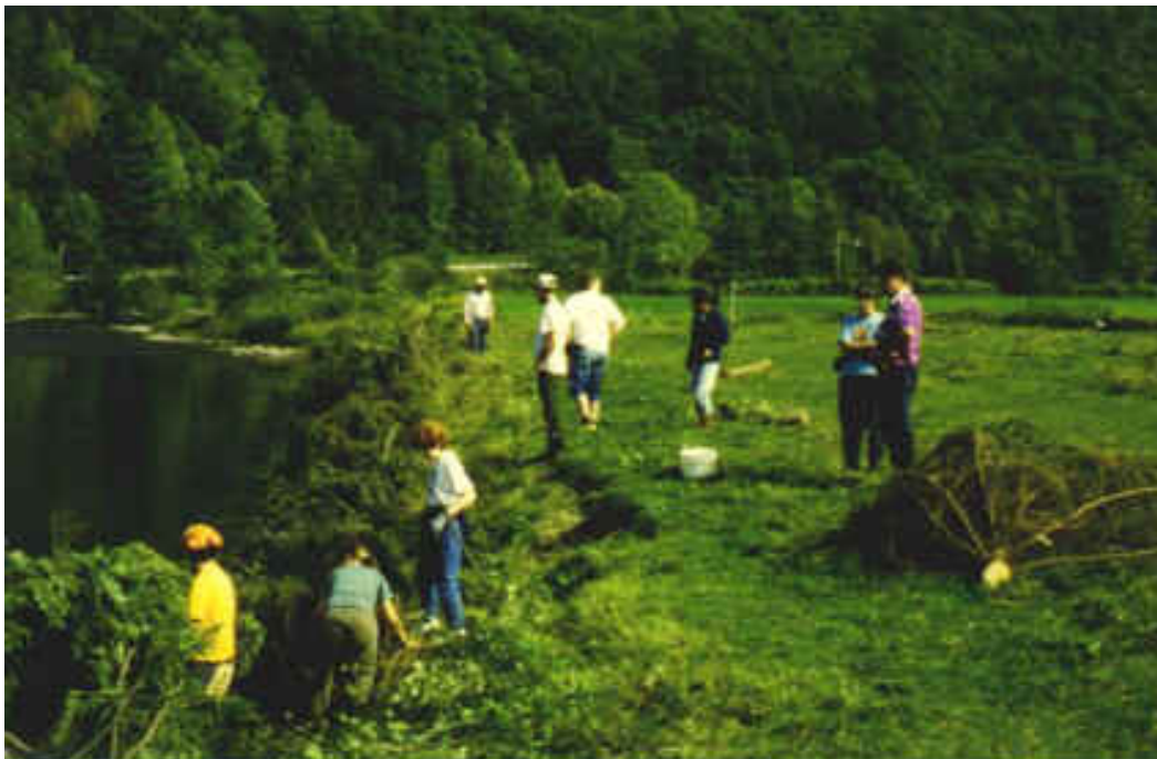
Installation of tree revetments
