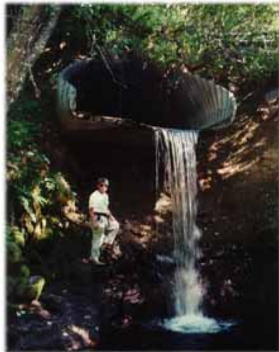
Upper basin culvert replacement for fish passage site.
