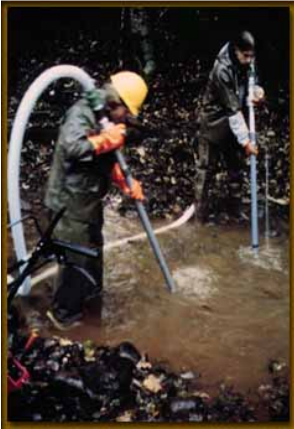
Americorps volunteers used water pumps and a suction dredge to remove fine sediment (sand) from spawning habitat of coho salmon.
