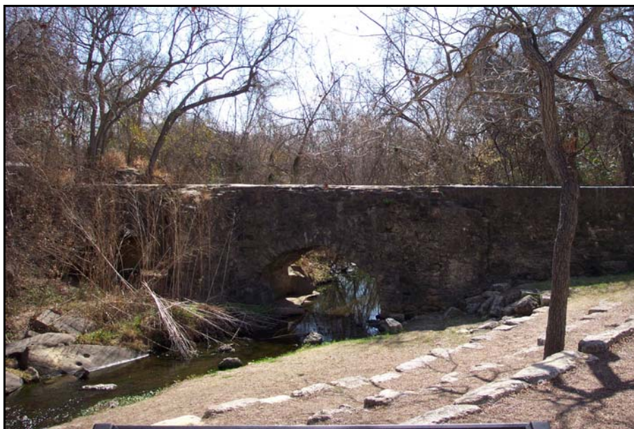
The Espada Aqueduct at SAAN Photograph by: Dan Cogan
