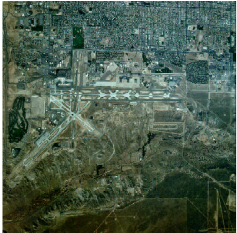
Figure 12: Sunport and KAFB runways north of the Tijeras Arroyo.
