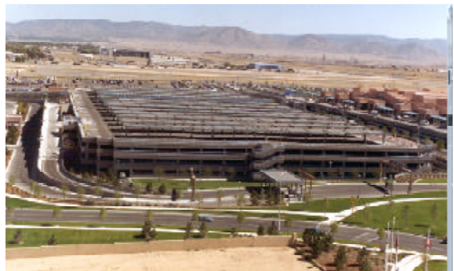
Figure 13: The International Sunport, New Mexico’s major air traffic hub and one of Albuquerque’s Specialty Activity Centers
