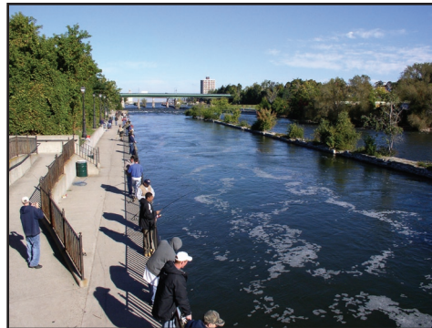
Varrick Dam North, Oswego River Photo Credit: U.S. EPA, GLNPO
