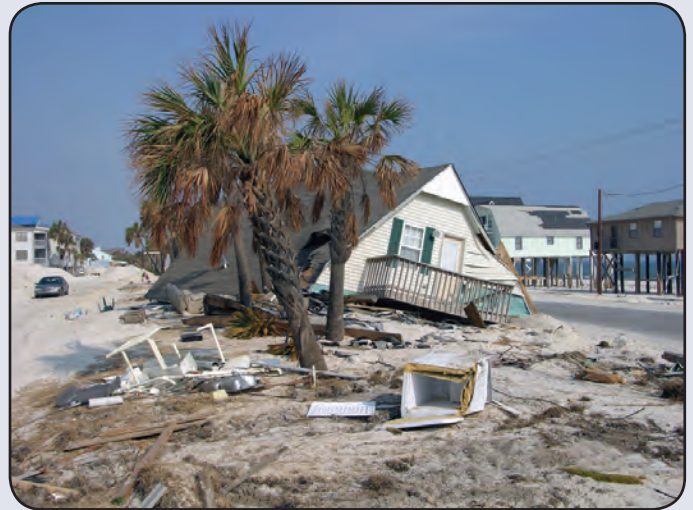
The aftermath of a hurricane
