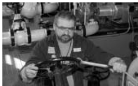
11. HIGH-SERVICE PUMPS send finished water from the WTF to the two water towers on site. Adjusting the flow rate of a high-service pump is Steve Barcelo.
