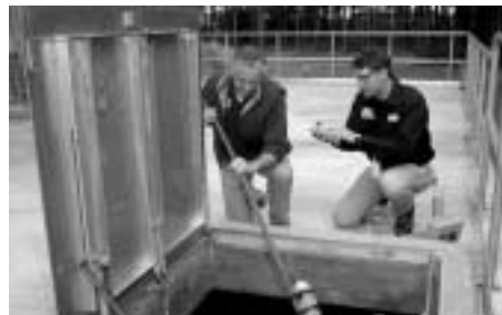
10. CLEAR WELL stores up to 250,000 gallons of what is now called "finished" water before its final chlorination and distribution. Seen taking a water sample at the clear well are Richard Lutz (left) and Jack Kulesa.
