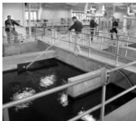
6. RETENTION TANK holds the water long enough to allow the chemicals time to react and form floc. To aid in the formation of floc, the water is then sent to a slow-mix tank. At the retention tank are: (from left) Steve Barcelo, Jack Kulesa (who is checking for floc particles), and Richard Lutz, plus Frank Masia.
