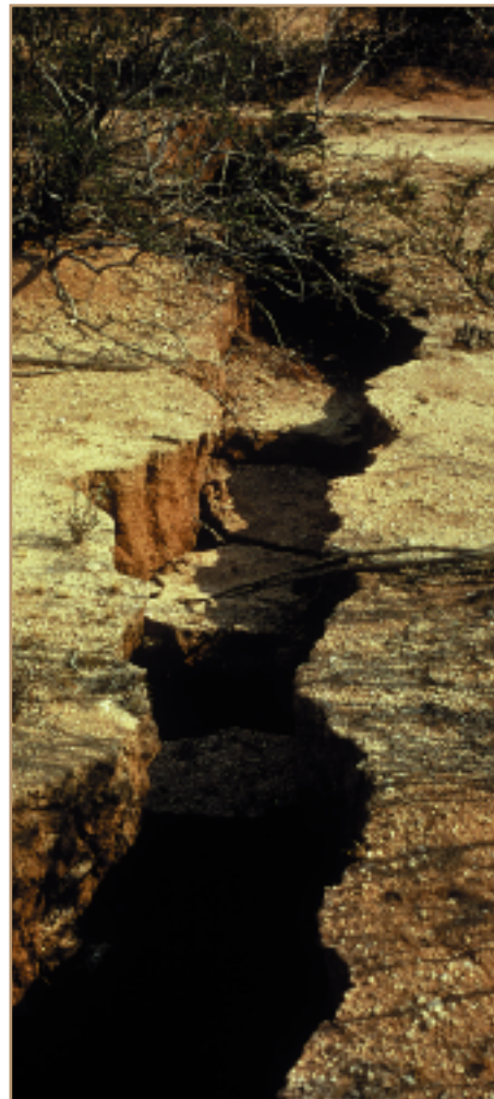
Figure 7. Earth fissure related to land subsidence, south-central Arizona.
