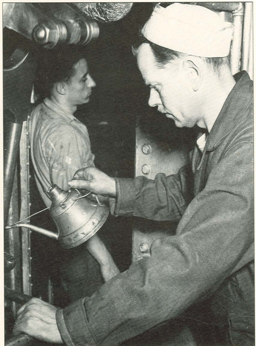
Left: Periodic supply runs meant replenishment of food for the crew and other items needed about the ship. Below: Engine-room duty never ended, only the watch schedule changed. An "oilcan jockey" lubricates the valve gear on Columbia River Lightship #93 as part of his duties.
