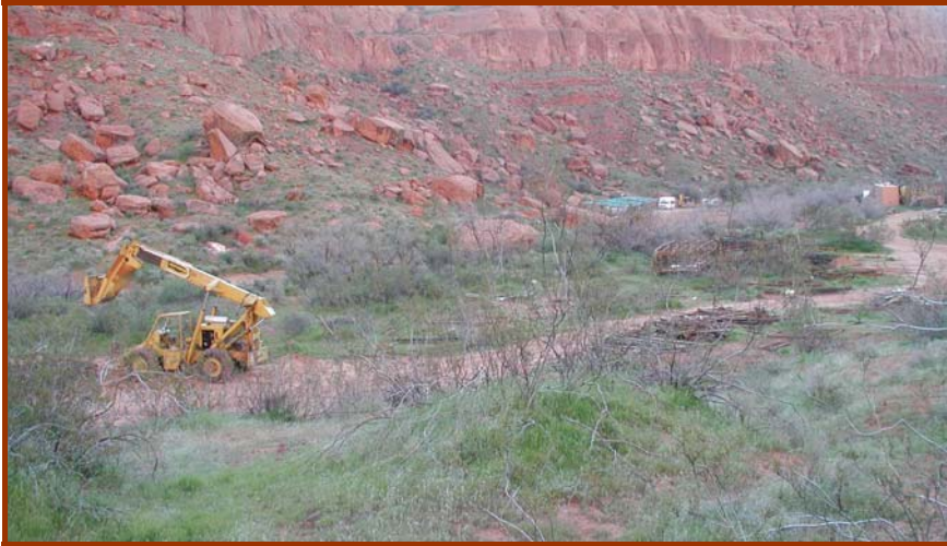
Photo 3. View of Tuacahn detention basin site, looking northwest.
