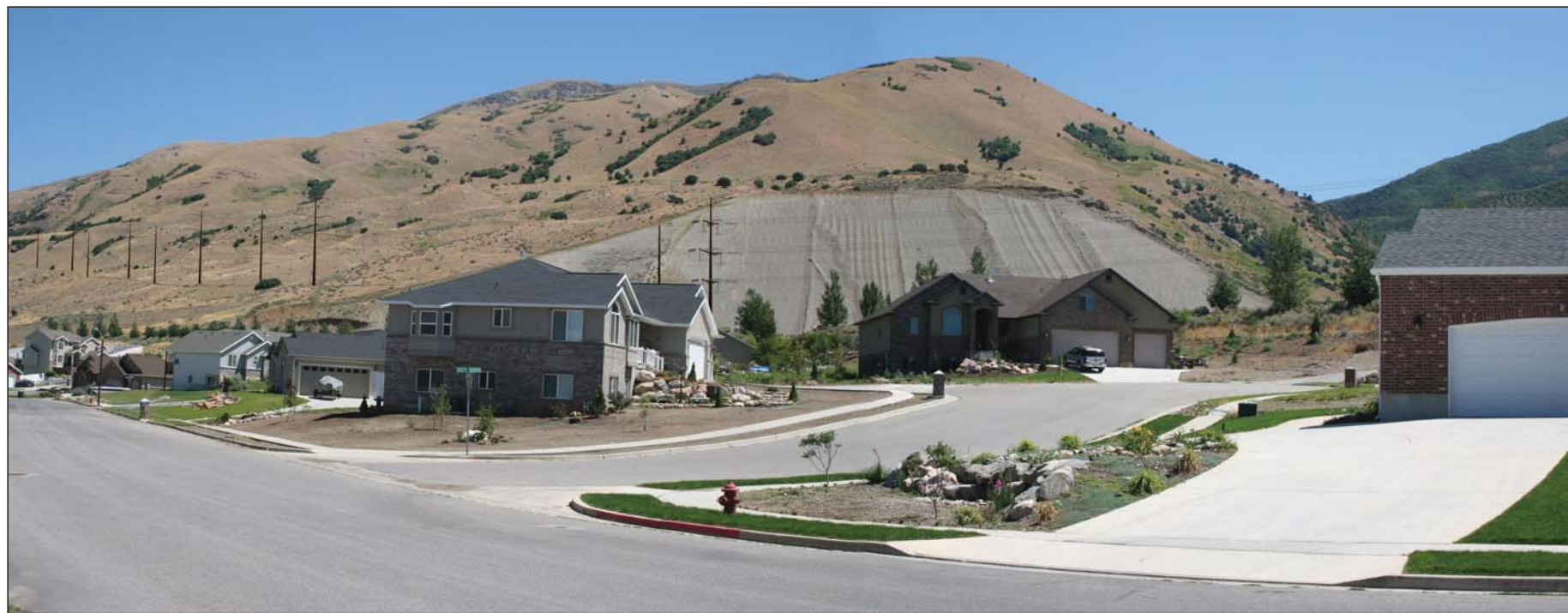
Simulation – Proposed 345kV transmission line and relocated 138kV transmission line in the foothills above Perry, Utah.
