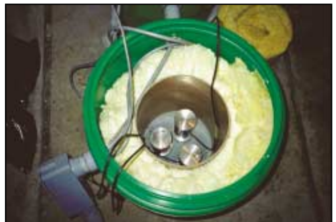
Figure 6. Polyurethane insulation in place.
