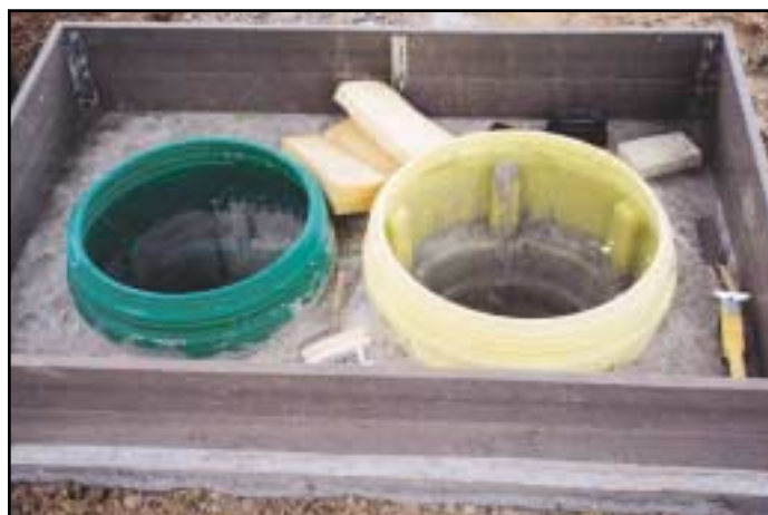
Figure 5. Vault door frame placed in concrete.
