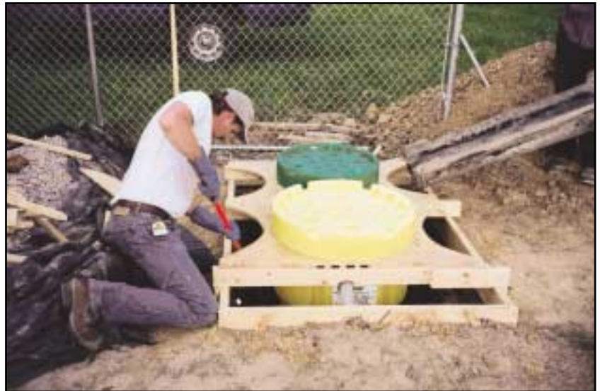
Figure 4. Placing concrete in excavated hole.
