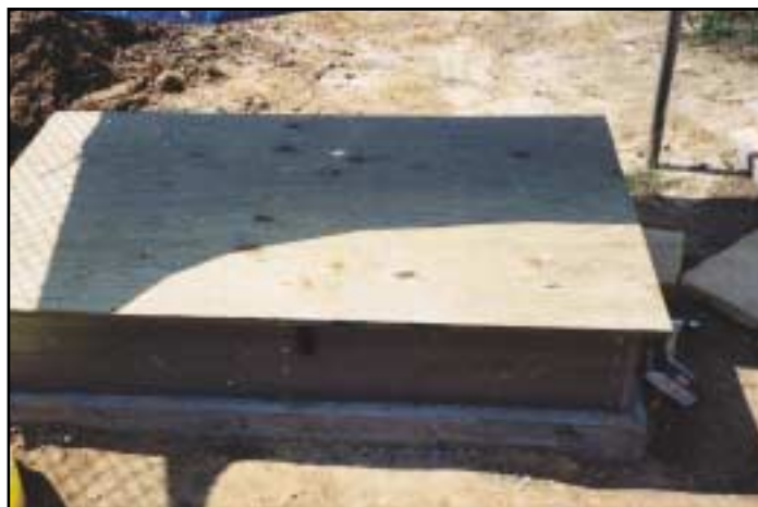
Figure 7. Vault door attached to frame.
