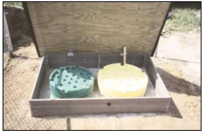
Figure 15. Vault construction and installation complete.
