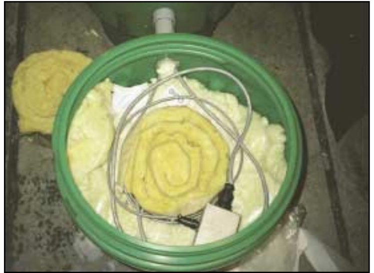
Figure 11. Insulation plug in place.
