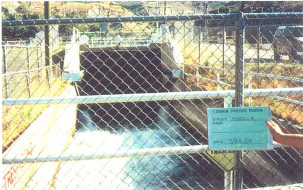
Photo 1-4. Murdock Diversion: upstream view of headworks canal.
