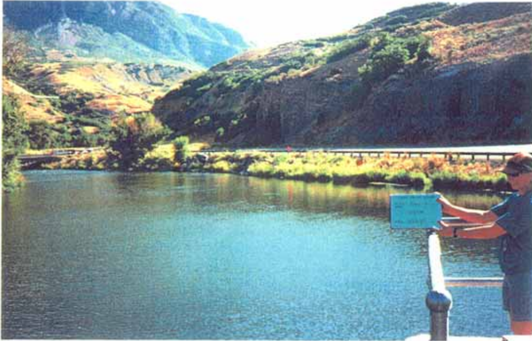
Photo 1-5. Murdock Diversion: channel upstream from structure.
