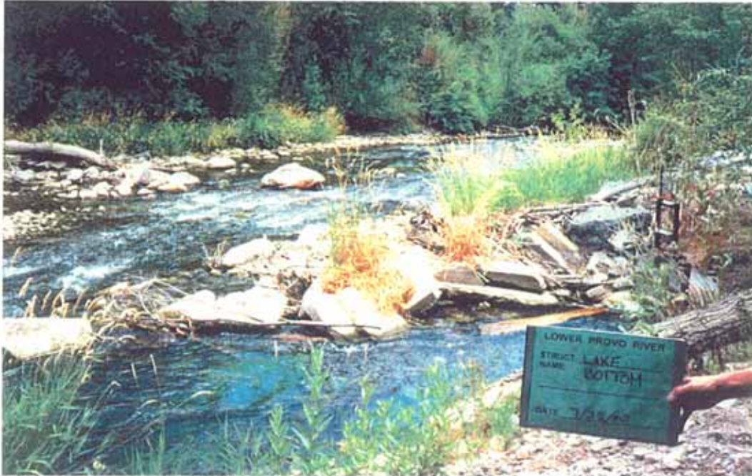
Photo 6-1. Lake Bottom Diversion: view of partial rock/rubble dam.
