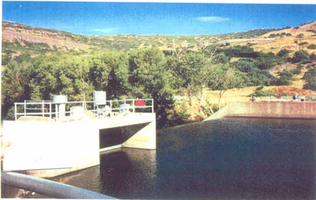
Photo 1-2. Murdock Diversion: view of structure and radial-gated sluiceway.
