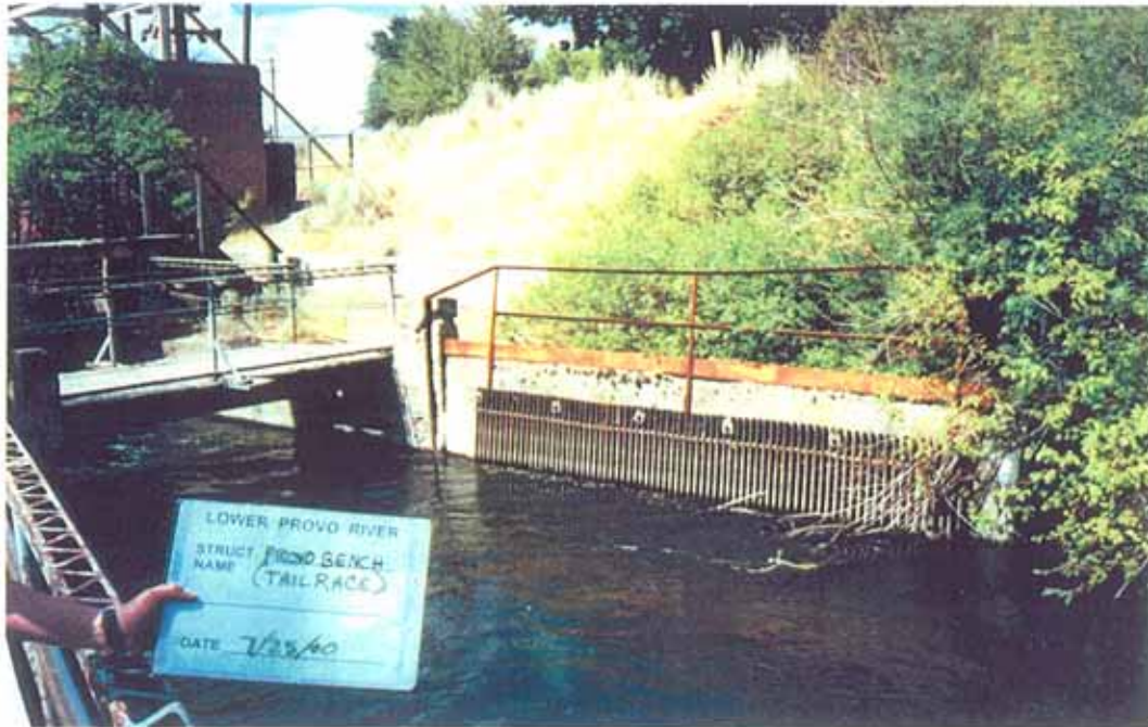
Photo 4-3. Provo Bench - diversion on tailrace: headworks to pumping station.
