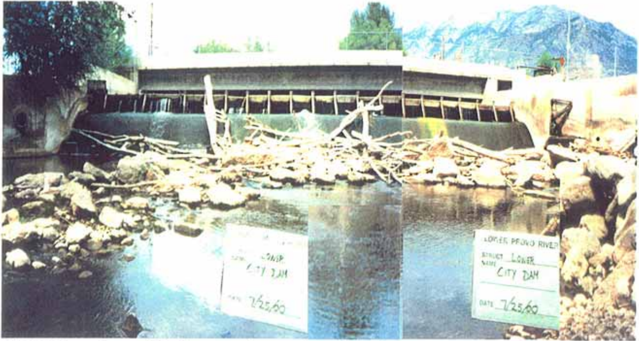
Photo 8-1. Lower City Dam: upstream view of structure.
