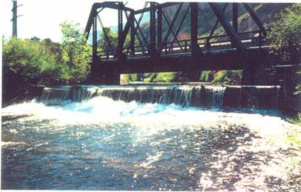
Photo 2-1. Timpanogos Diversion: upstream view.
