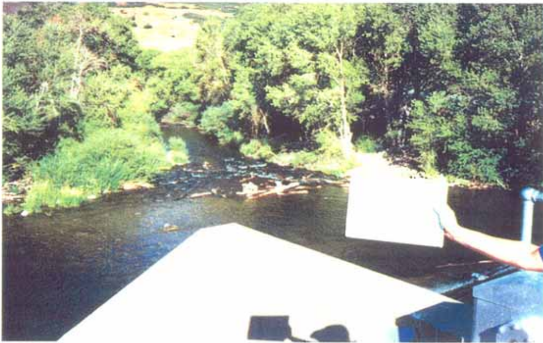
Photo 1-6. Murdock Diversion: channel downstream from structure.
