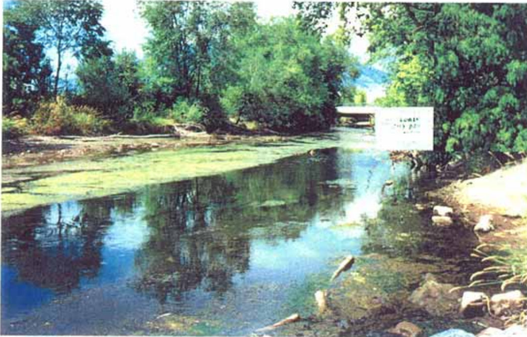
Photo 8-5. Lower City Dam: view of channel upstream from structure.
