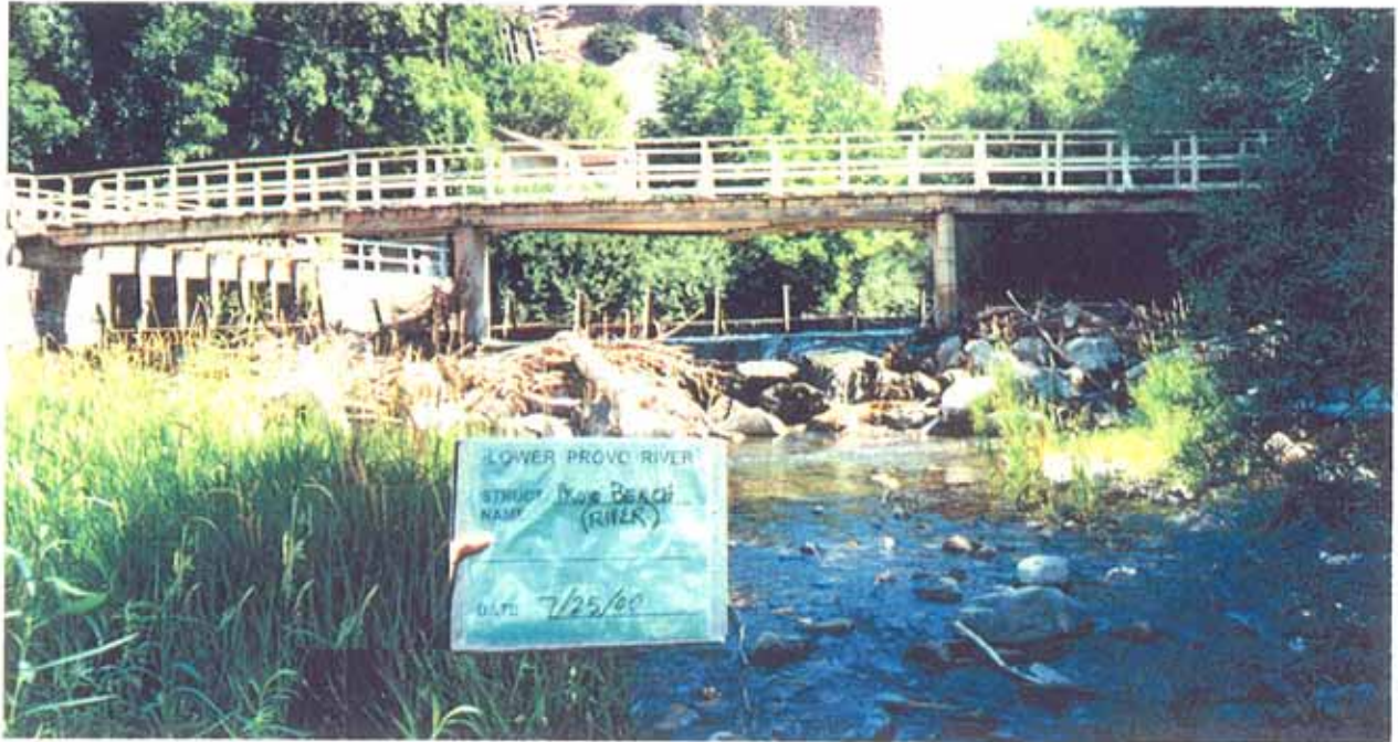
Photo 3-1. Provo Bench - diversion on river: upstream view of structure.
