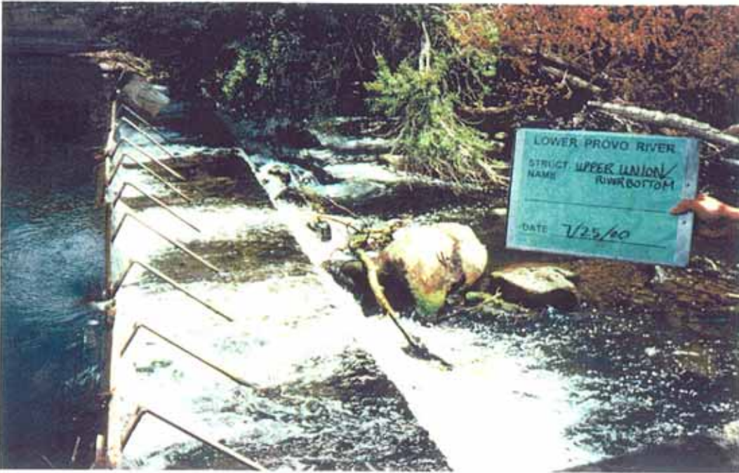
Photo 5-3. Upper Union Diversion: kick-leg dam structure.
