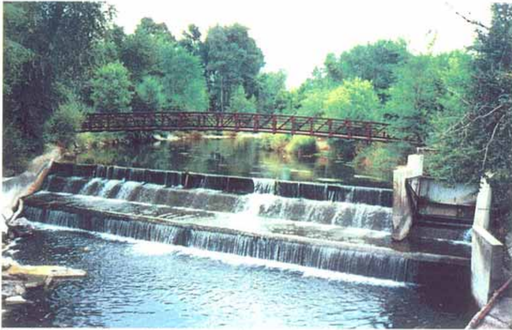
Photo 7-1. Upper City Dam: upstream view of structure.
