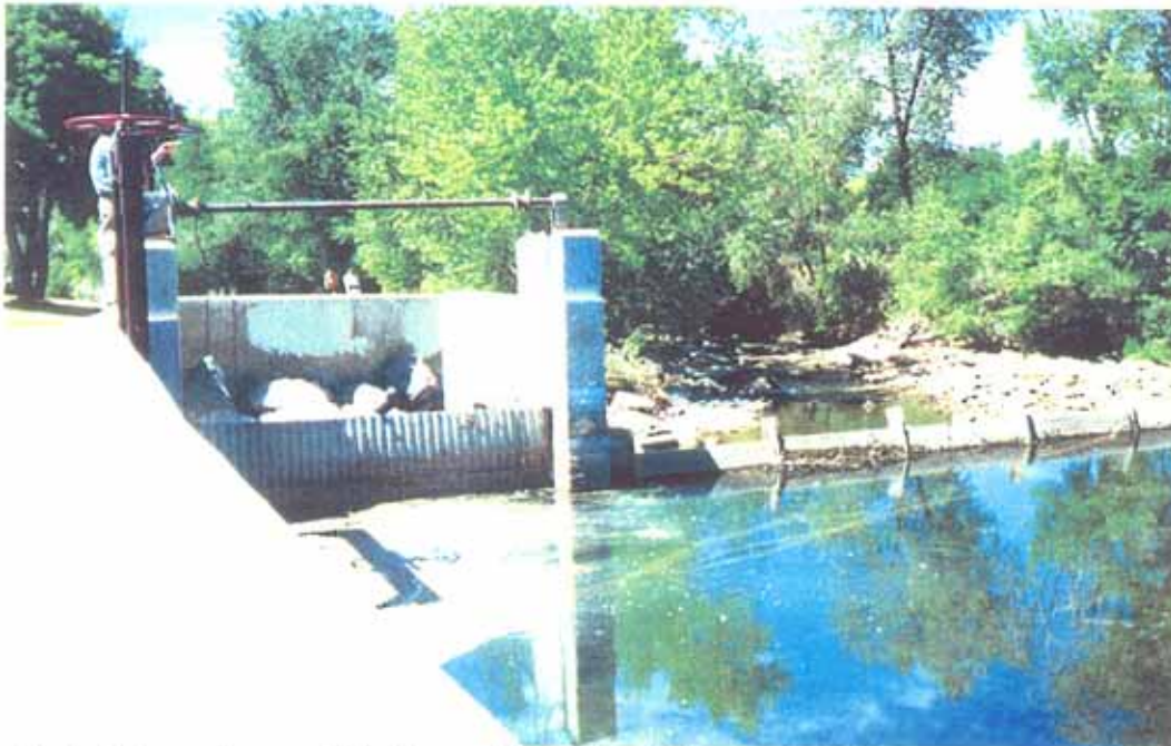
Photo 8-4. Lower City Dam: view of radial-gated sluiceway.
