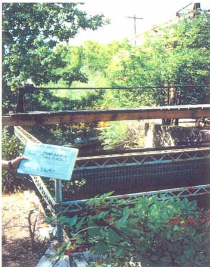
Photo 4-2. Provo Bench - diversion on tailrace: canal headworks.
