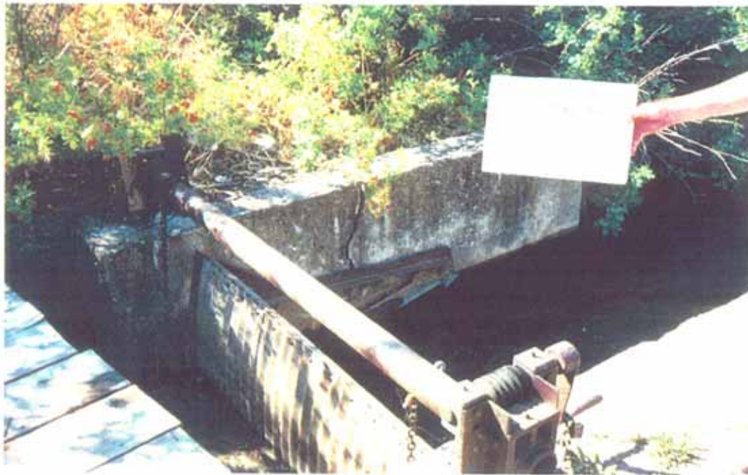
Photo 2-4. Timpanogos Diversion: canal headworks.
