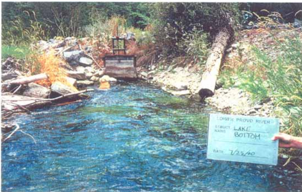
Photo 6-2. Lake Bottom Diversion: canal headworks.
