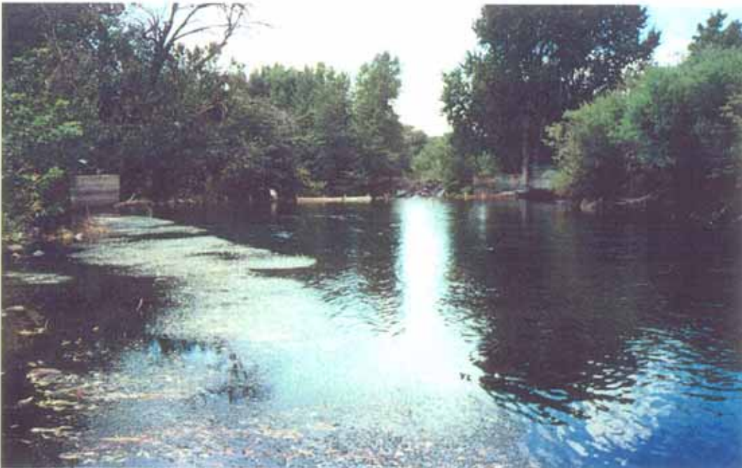
Photo 5-2. Upper Union Diversion: downstream view of structure.
