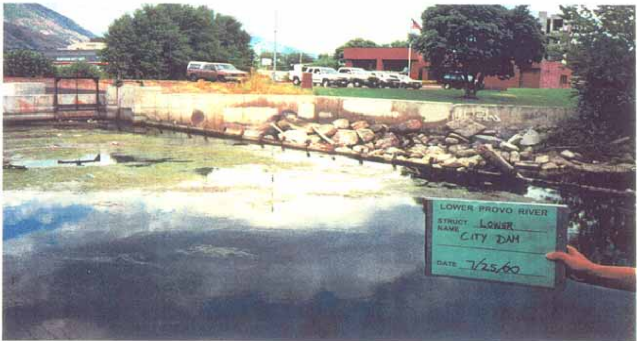
Photo 8-2. Lower City Dam: downstream view of structure.
