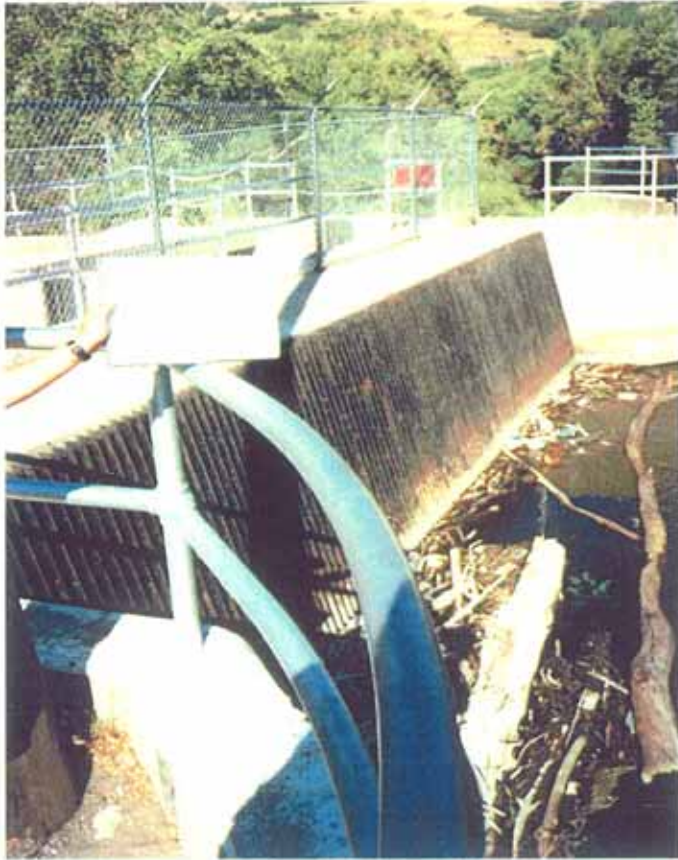
Photo 1-3. Murdock Diversion: grate at canal headworks.
