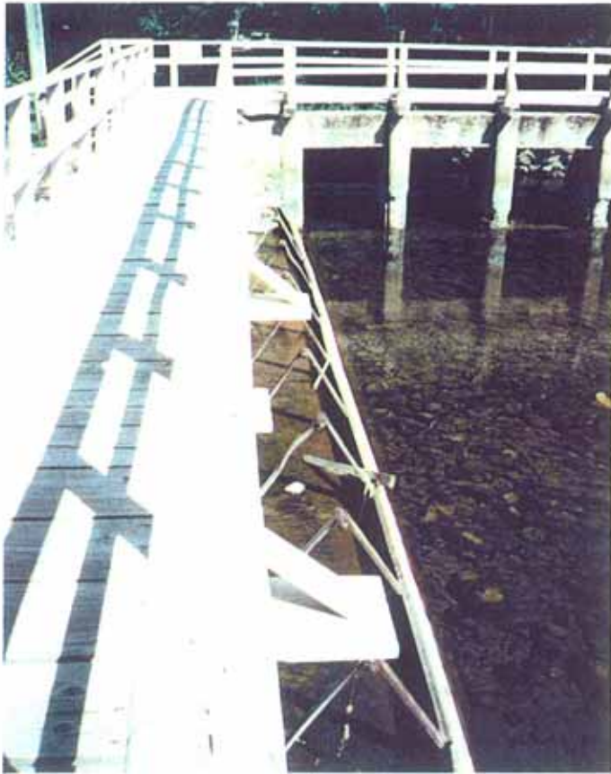
Photo 3-3. Provo Bench - diversion on river: kick-leg dam structure.
