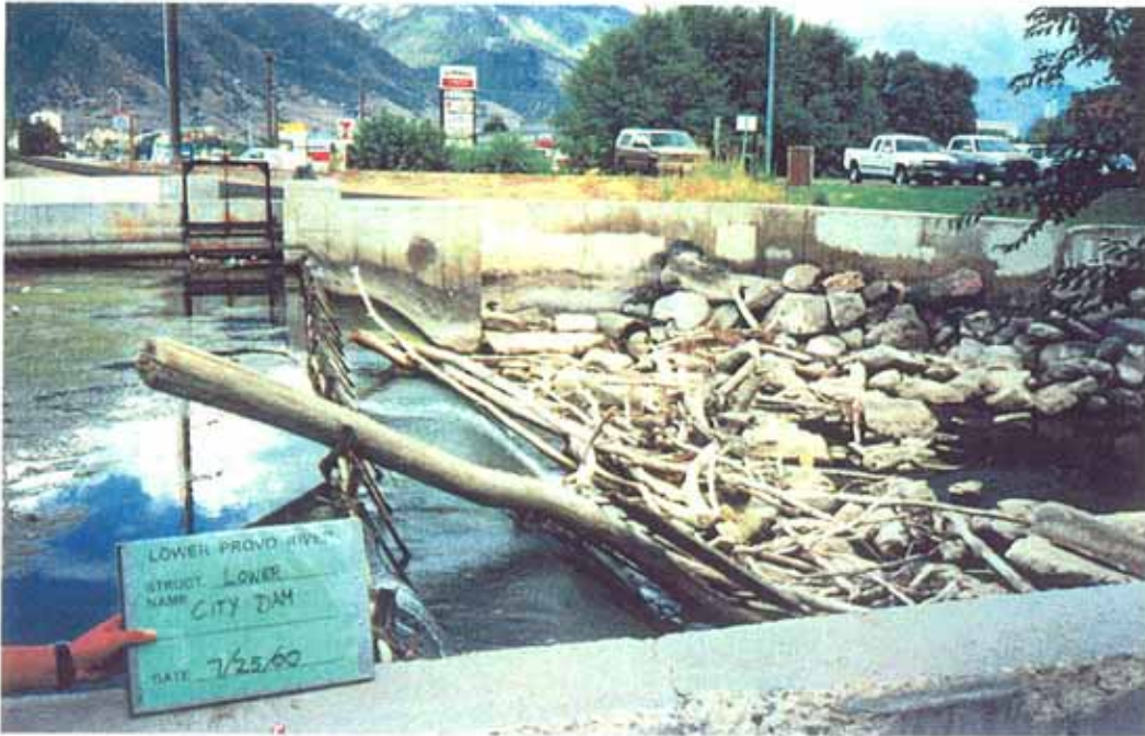
Photo 8-3. Lower City Dam: view of kick-leg structure and canal headworks.
