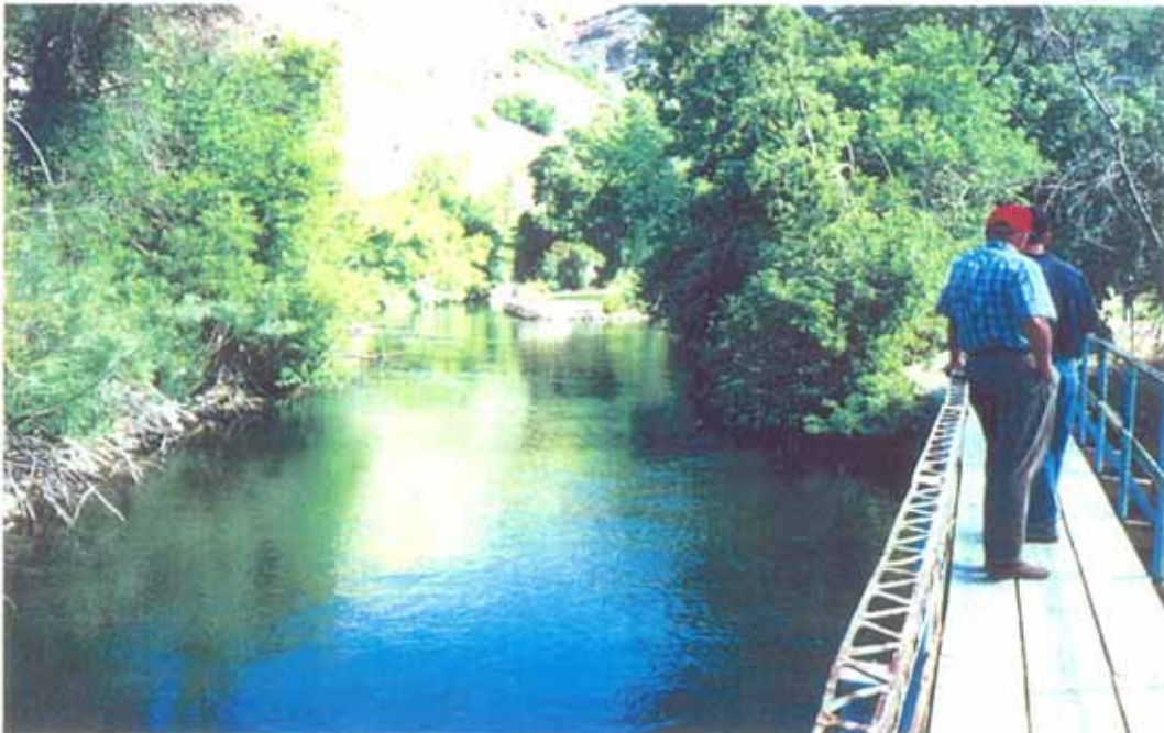
Photo 4-4. Provo Bench - diversion on tailrace: view of tailrace above structure.
