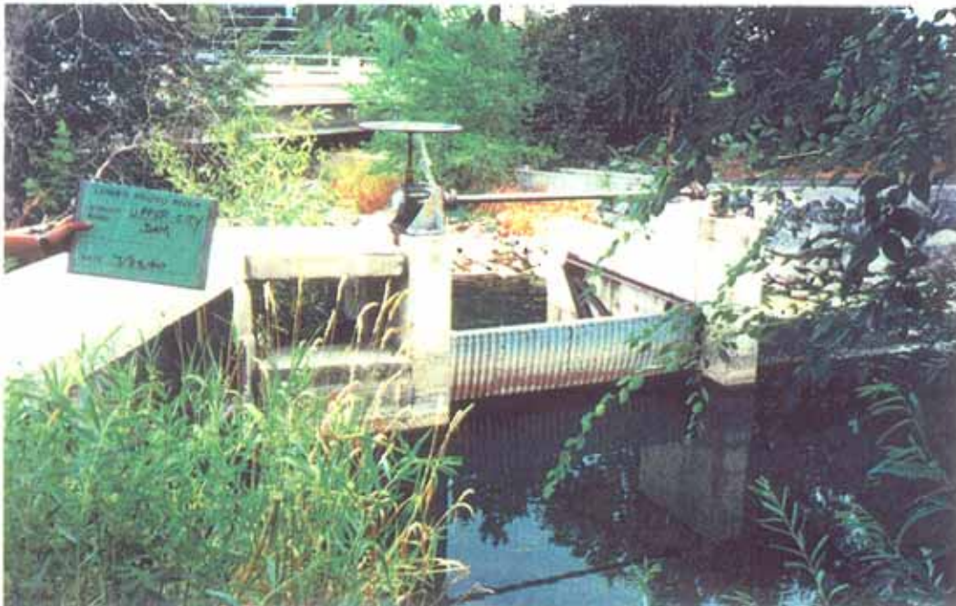
Photo 7-4. Upper City Dam: radial gated sluiceway.
