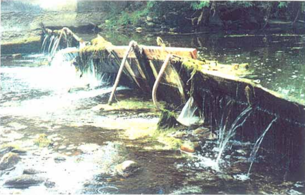
Photo 9-3. Fort Field Diversion: kick-leg structure.
