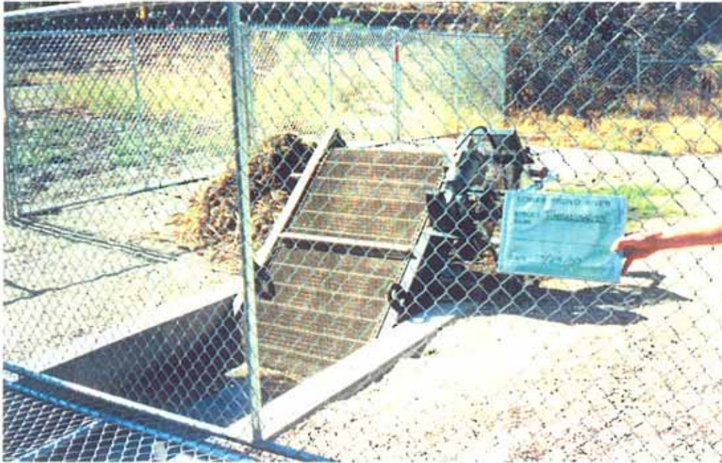
Photo 2-5. Timpanogos Diversion: mechanical moving fish screen at pipe entrance.
