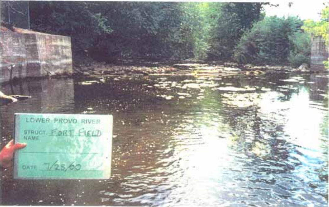
Photo 9-2. Fort Field Diversion: downstream view of structure.
