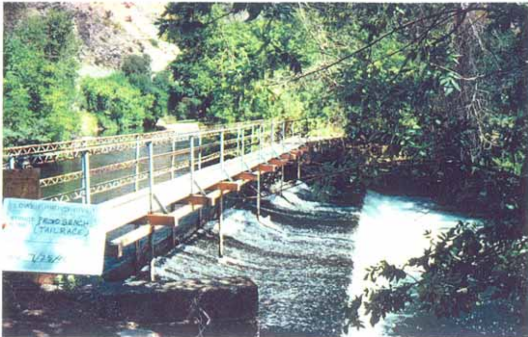
Photo 4-1. Provo Bench - diversion on tailrace: flashboard and concrete structure.
