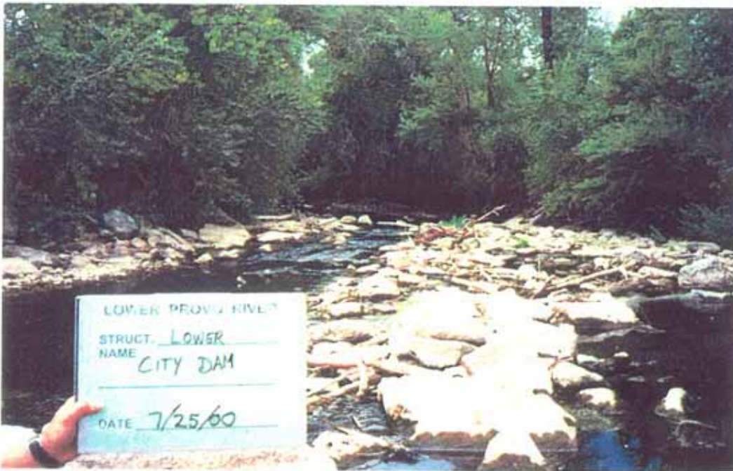
Photo 8-6. Lower City Dam: view of channel downstream from structure.
