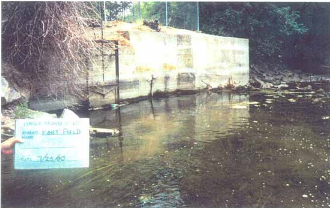
Photo 9-4. Fort Field Diversion: canal headworks.
