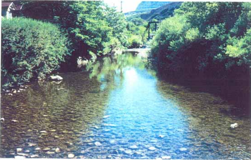
Photo 3-5. Provo Bench - diversion on river: channel upstream from structure.
