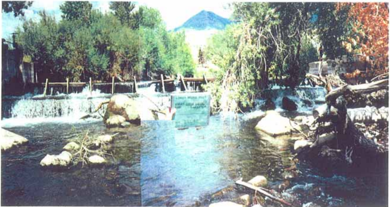
Photo 5-1. Upper Union Diversion: upstream view of structure.
