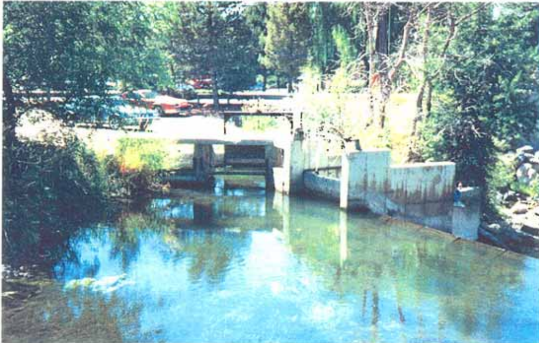
Photo 7-3. Upper City Dam: headworks to Lower East Union/Factory Race canals.
