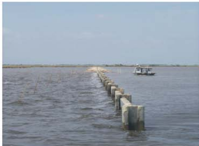
Concrete "H" pile/panel structures, similar to this one, will be installed at locations within the project area where shoreline erosion is critical. Soils with high amounts of organic material, which have poor strength, necessitated the use of a structure such as this.
