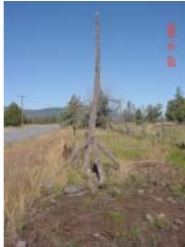
Figure 3-11. Photo of telephone pole built along Willow Valley Road. (Photo by Robert Mutch, 2002.)
