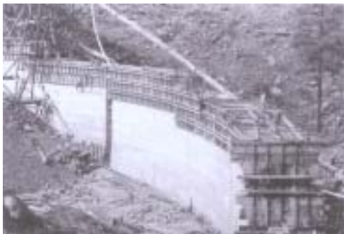
Figure 4-5. Construction of Gerber Dam.
