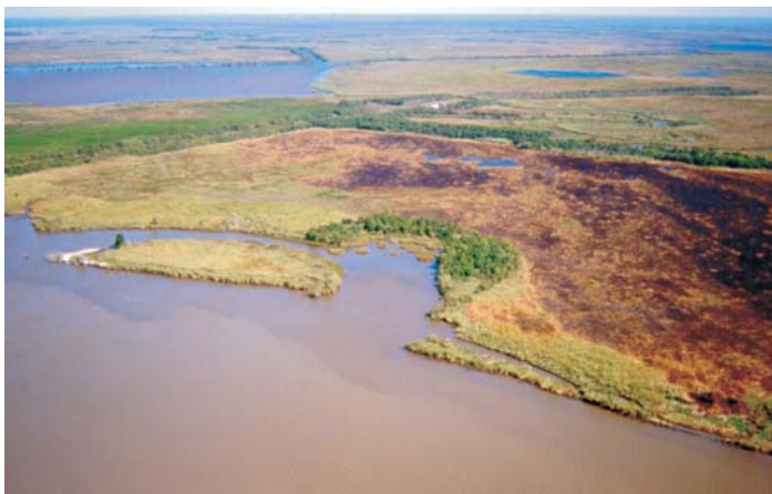
Pre-construction, facing east toward Onion Lake.
