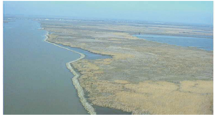
Post-construction, facing northeast towards Onion Lake.
