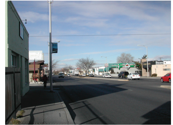
Signalized intersections that are spaced too far apart result in unprotected, mid-block crossings
