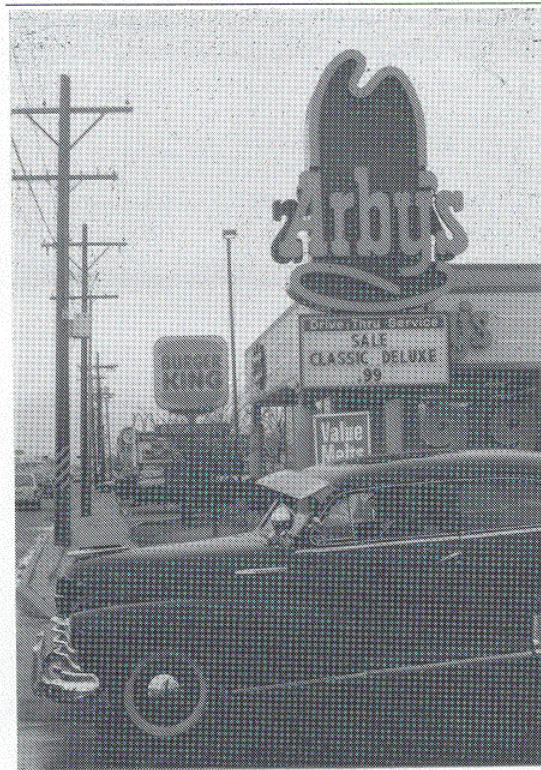
Strip commercial on Fourth Street, south of Montaña Road.
