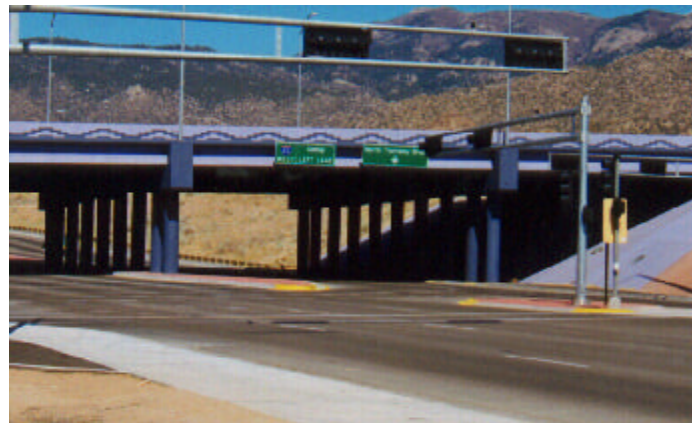
Tramway Blvd. underpass at I-40.
