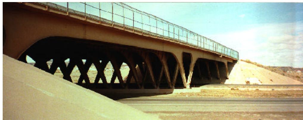
Unser Blvd. Bridge
