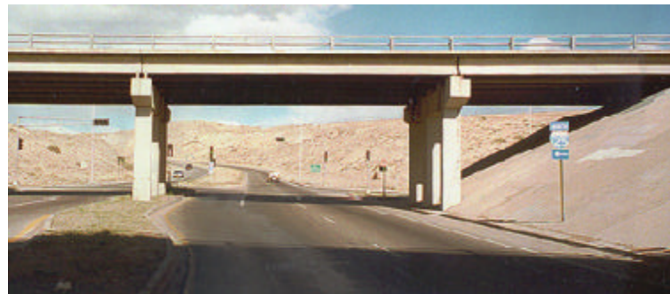
I-25 Bridge looking east.
