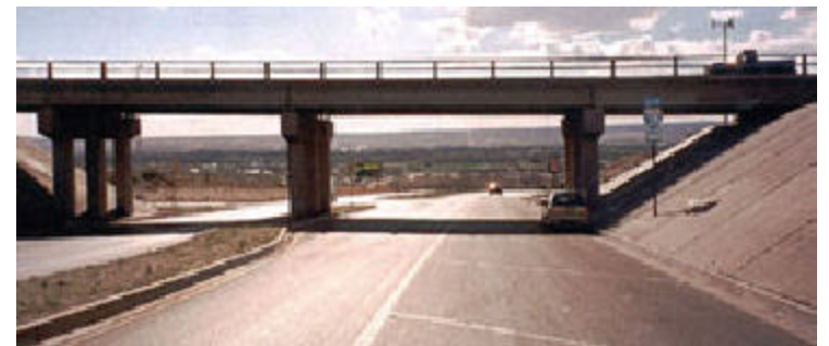
I-25 bridge looking west.
