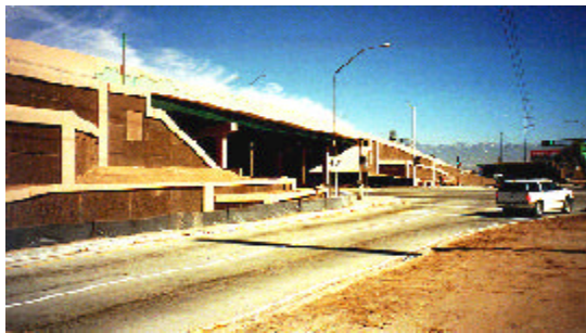
Rio Grande Bridge and Planting Terraces.
