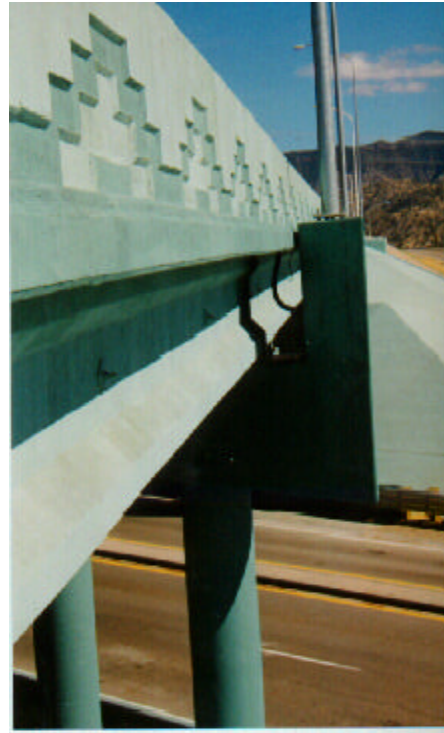
I-40 over Central Ave.
