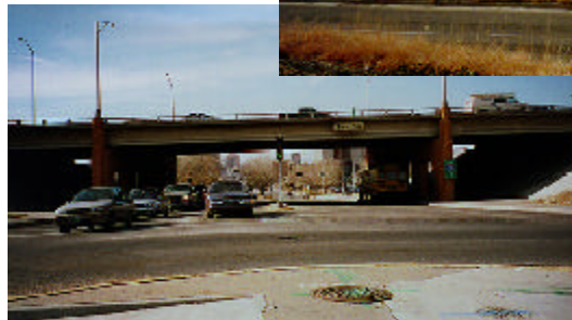
Martin Luther King Jr. Bridge
