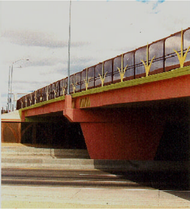
Wyoming Blvd. Bridge at I-40.
