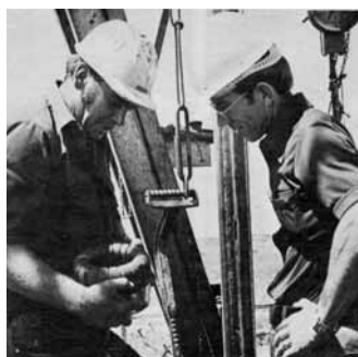
WORKERS examine the diamond bit used for cutting cores. The drilling went to 800-plus meters so that the underlying salt beds could be evaluated.
