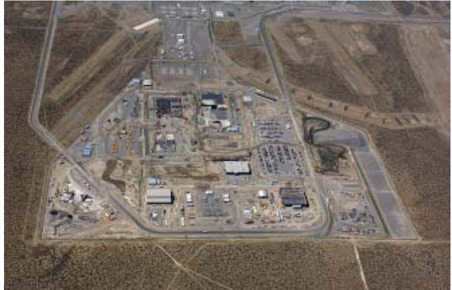
Aerial view of the Waste Treatment Plant construction site.
