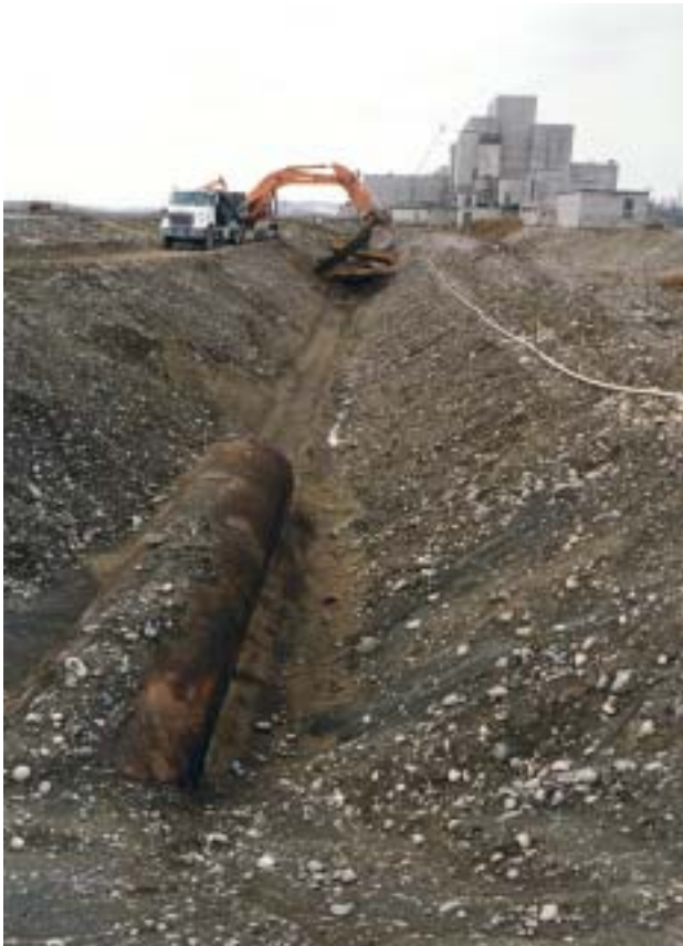
Digging up reactor effluent cooling water piping and surrounding contaminated soil.
