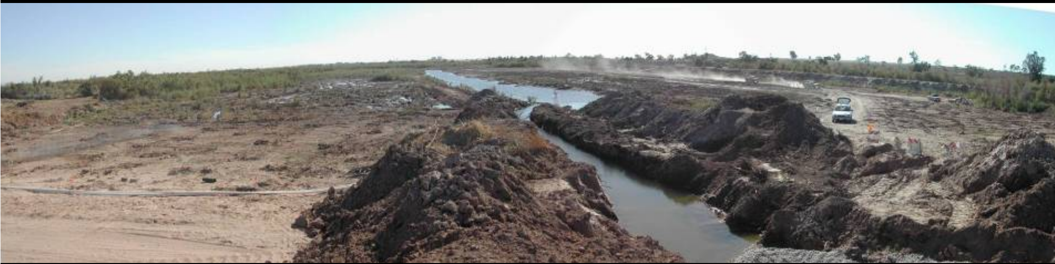
THE IBIS LAKE MARSH AREA DURING CHANNEL EXCAVATION, NOVEMBER 2005.
