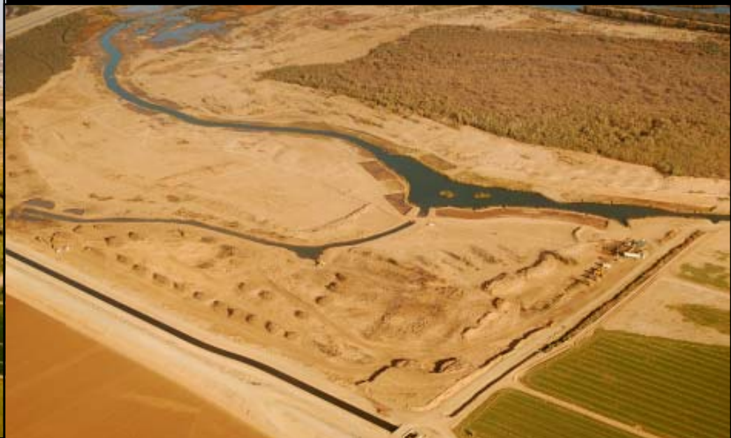
YEW AFTER CLEARING AND CHANNEL EXCAVATION 2006
