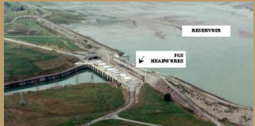
Pump Generating Station
