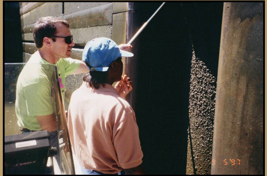
Kerr Lock and Dam (COE), Tulsa OK
