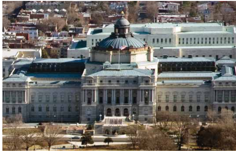
The Library of Congress underwent a number of renovations that improved visitor services, restored historic architectural features, and enhanced systems to protect its heritage assets.
