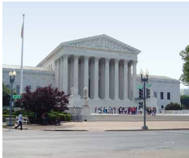
Significant progress has been made towards achieving the goal of replacing nearly all the original electrical, plumbing, heating, ventilating, and HVAC systems throughout the Supreme Court building.
