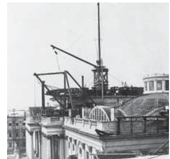
Since its inception, the Capitol has continued to evolve, including the addition of its iconic cast-iron dome in the 19th Century.
