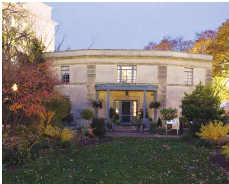
The AOC has begun a phased approach toward modernizing the USBG administration building while maintaining its historic appearance.
