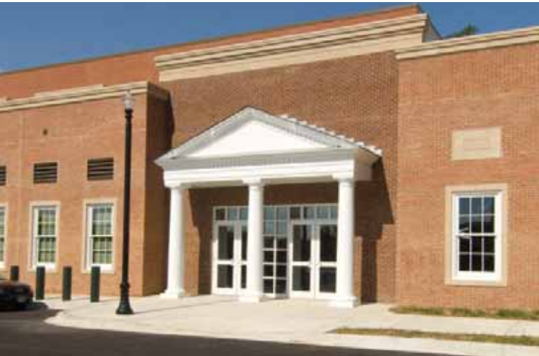
The AOC is responsible for the maintenance, care, and operation of the buildings, grounds, and security enhancements of the United States Capitol Police.
