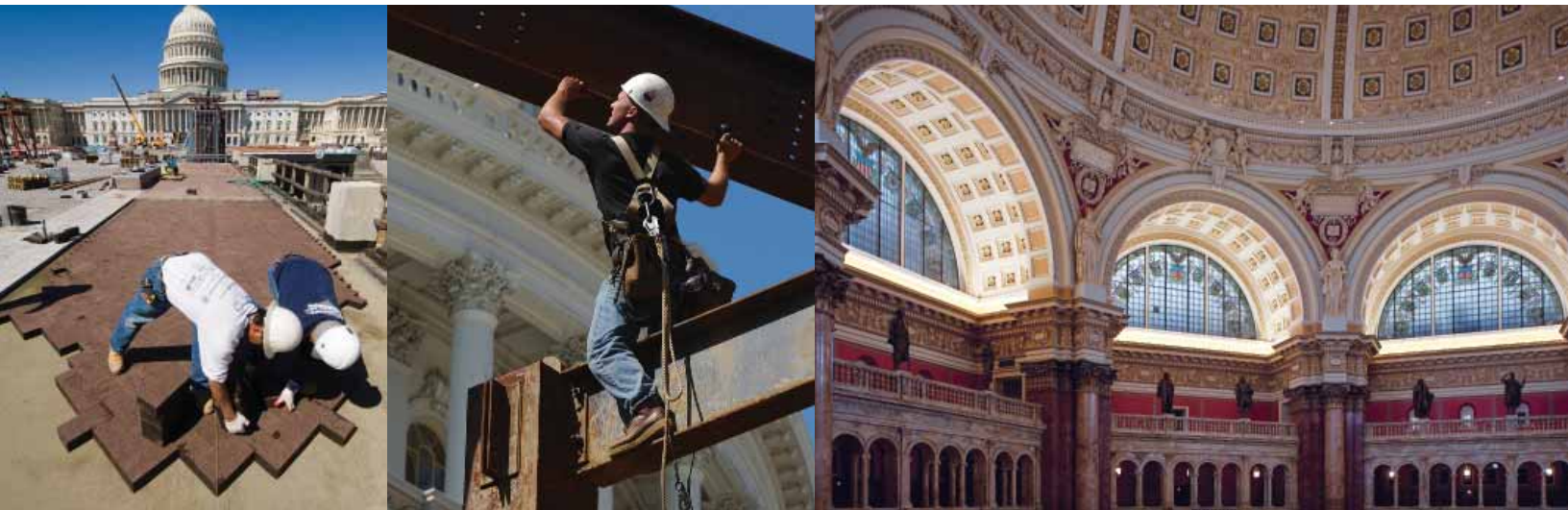
The AOC plays an important role in construction and restoration activities that took place in and around the Capitol, such as those in conjunction with the creation of the Capitol Visitor Center and the historic arch restoration in the Thomas Jefferson Building's Main Reading Room.
