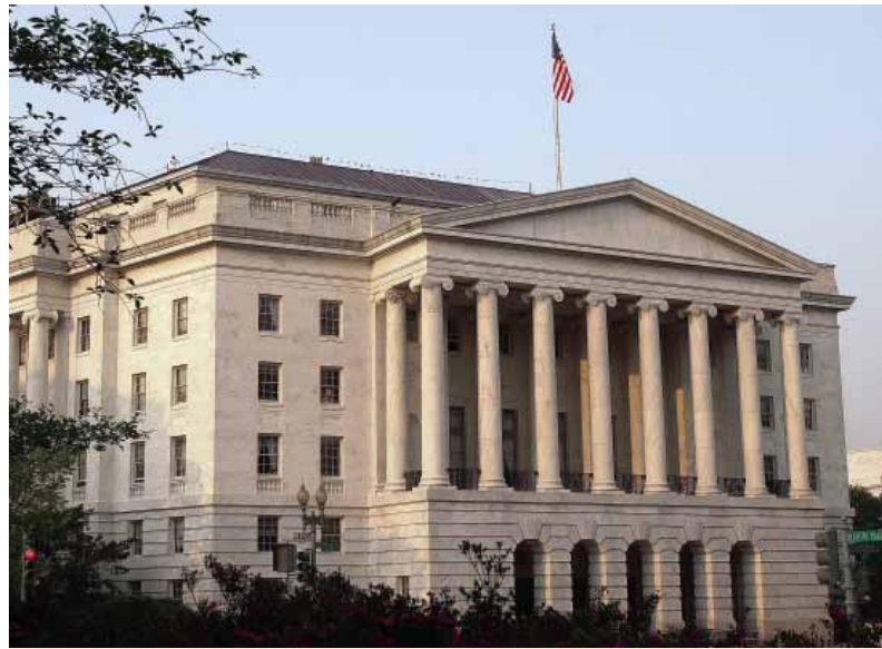
In 2008, the HOB completed 116 construction and renovation projects, including the renovation of the third floor of the Longworth House Office Building.
