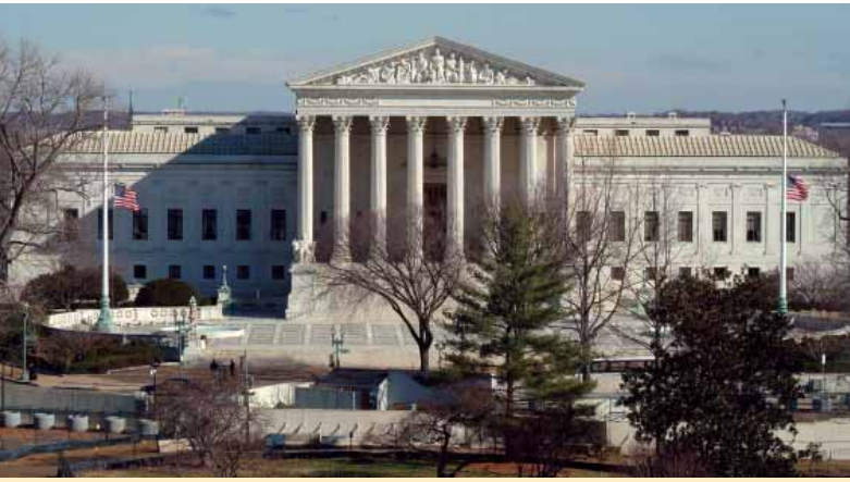
The ongoing Supreme Court modernization project included landscape and hardscape renovations as well as safety improvements.
