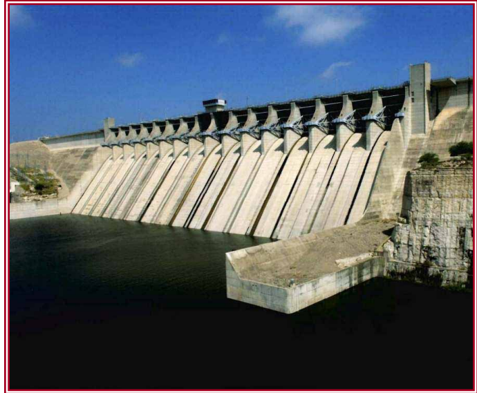
Amistad Storage Dam
