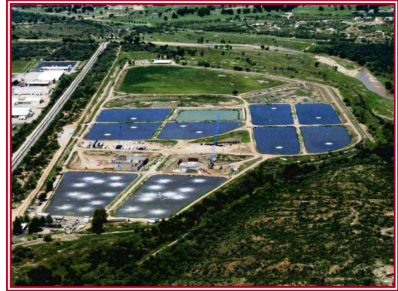
Nogales Int'l Wastewater Treatment Plant
