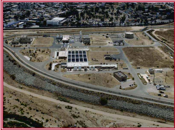
South Bay Int'l Wastewater Treatment Plant
