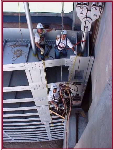
Falcon Storage Dam
