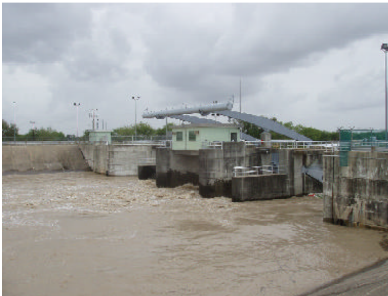
High flow passes through Retmal Dam
