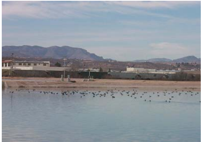
Nogales International Wastewater Treatment Plant
