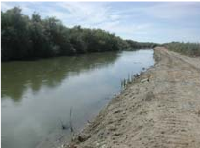
Wellton-Mohawk Bypass Drain
