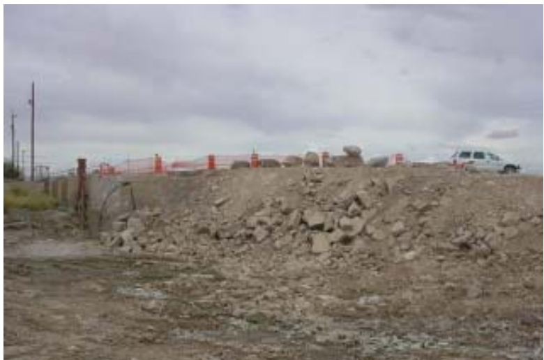
Work at Riverside Dam
