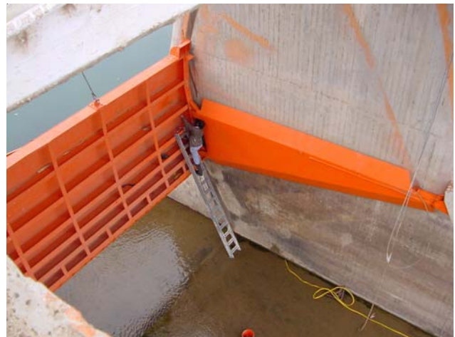
Morelos Dam maintenance
