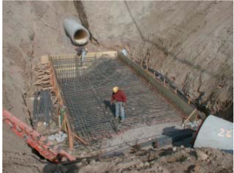
Work on the Primary Effluent Return Connection
