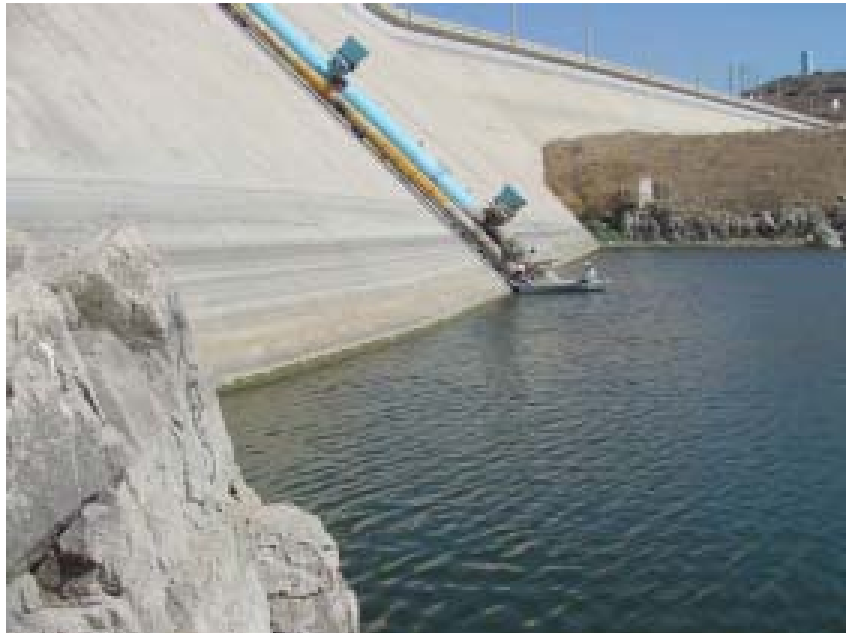
Installation of a telemetry system at Rodriguez Dam
