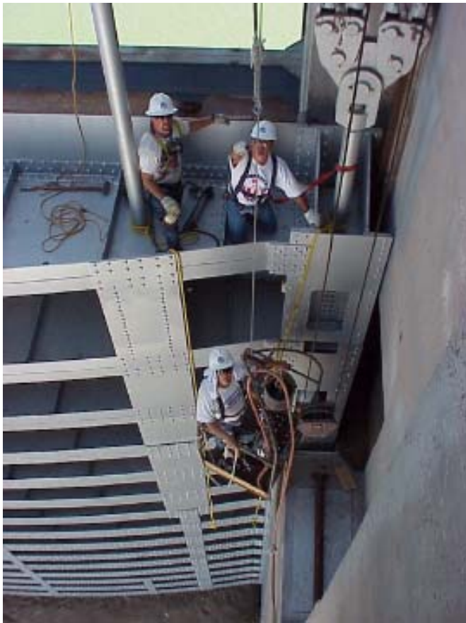
Falcon Dam spillway gate
