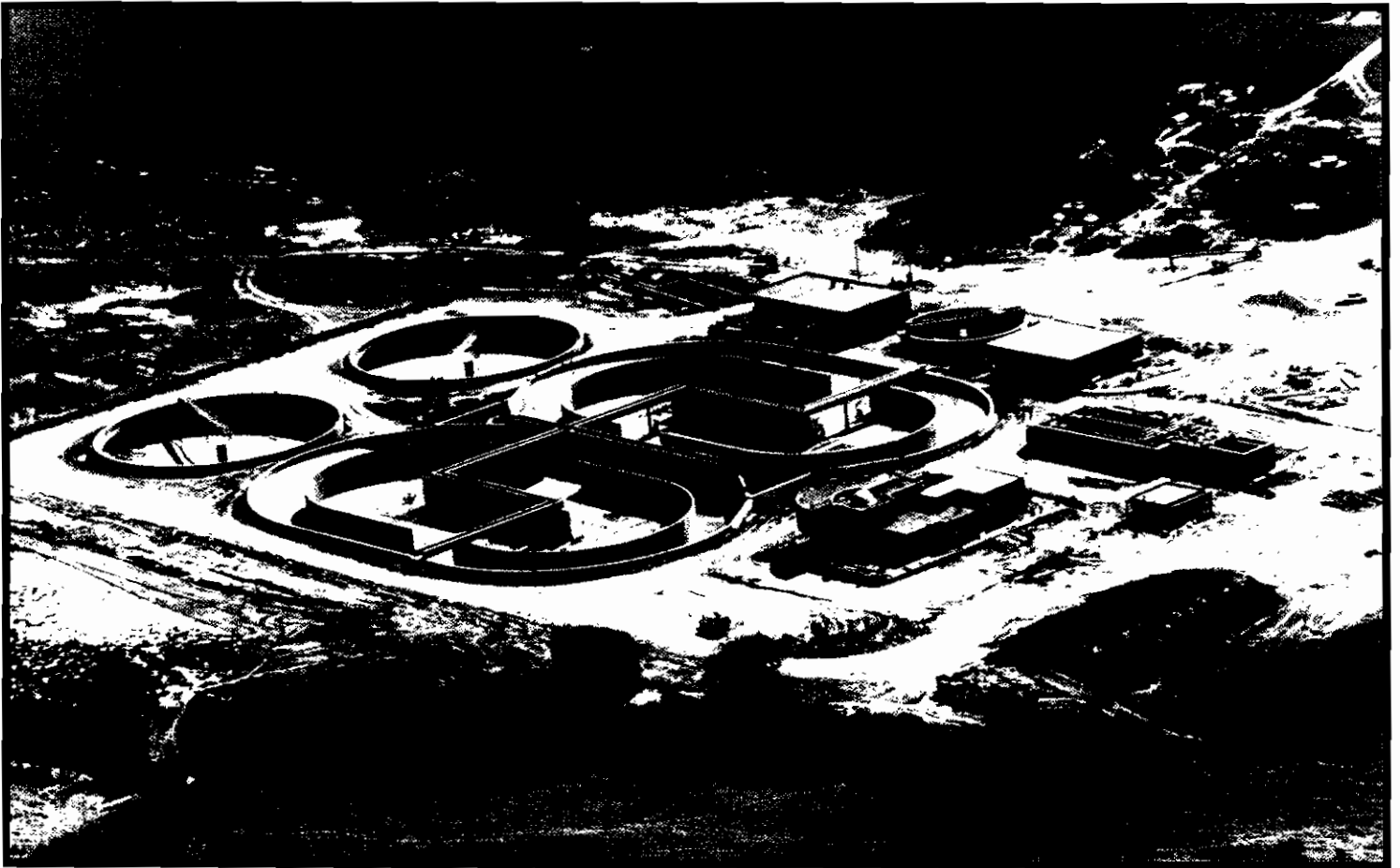
Wastewater Treatment Plant at Piedras Negras City, Coahuila.
