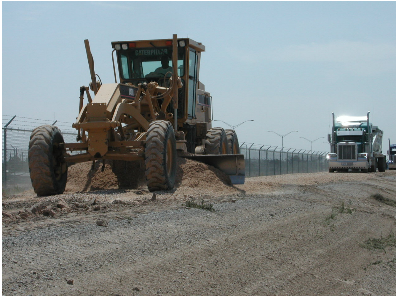
Placement of surfacing material
