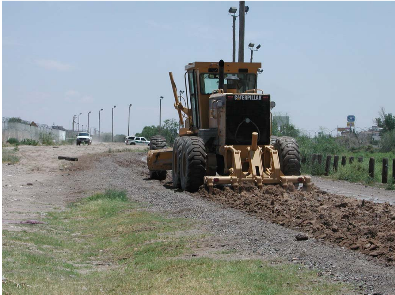
Scraping top of levee road
