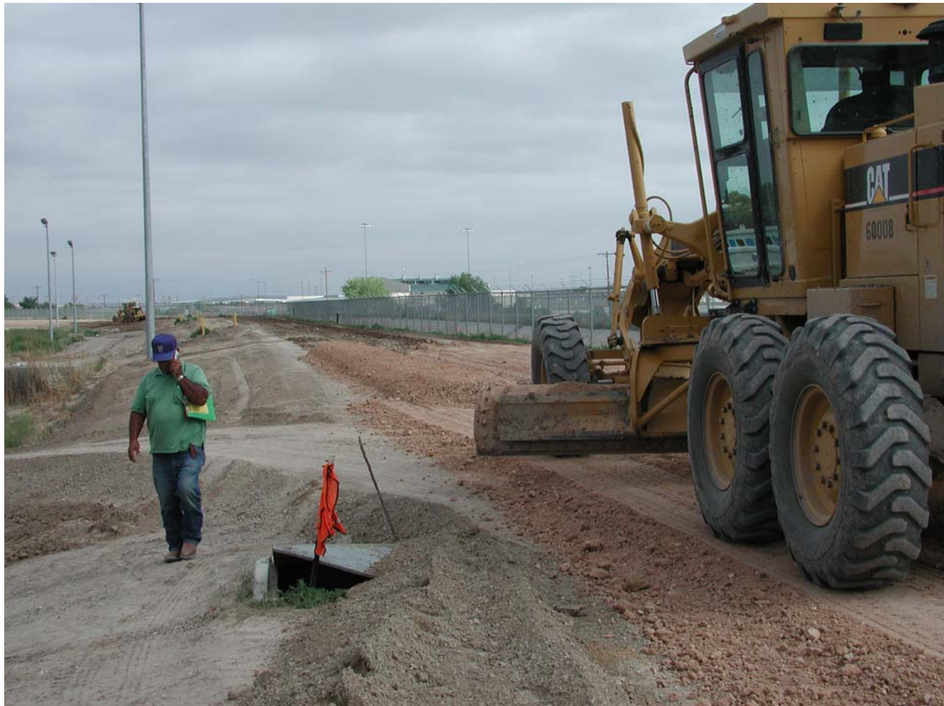
Placement of embankment material
