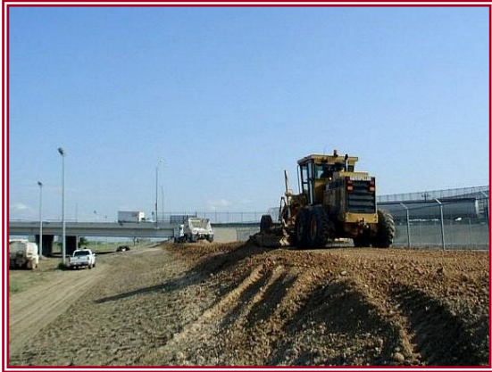
Upper Rio Grande Levee Improvements
