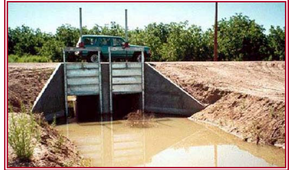
Rio Grande Wasteway at Mesilla
