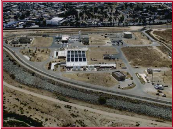
South Bay Int'l Wastewater Treatment Plant
