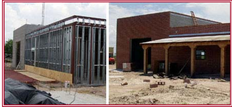
Anzalduas Administration & Maintenance Building
