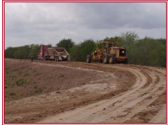
Lower Rio Grande Levee Improvements
