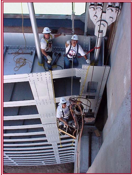
Falcon Storage Dam
