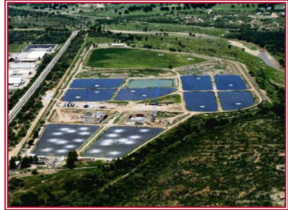
Nogales Int'l Wastewater Treatment Plant
