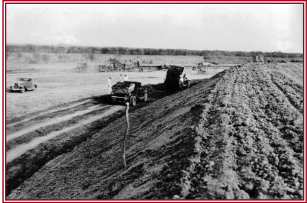
Lower Rio Grande U.S. Main Floodway
